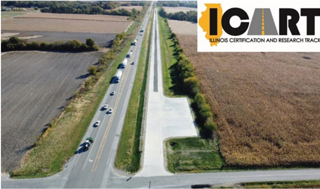
Figure 2. Photo. Aerial photograph of ICART.
