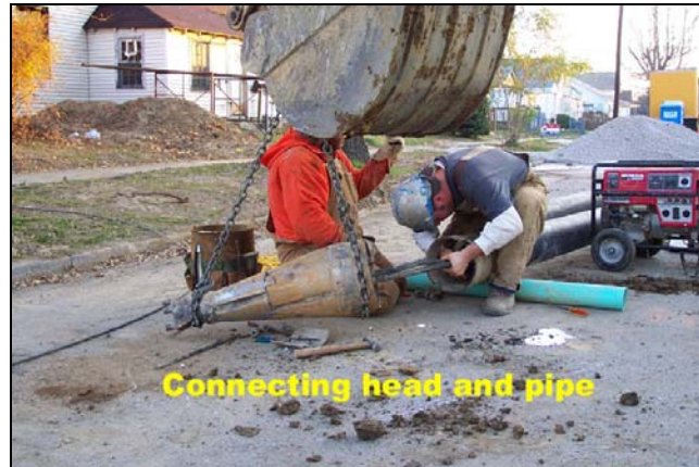
Figure 2.66 Connection of bursting head and pipe
