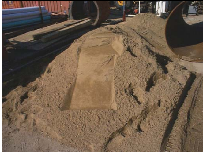
Figure 4.13 Soil excavated from the bore hole
