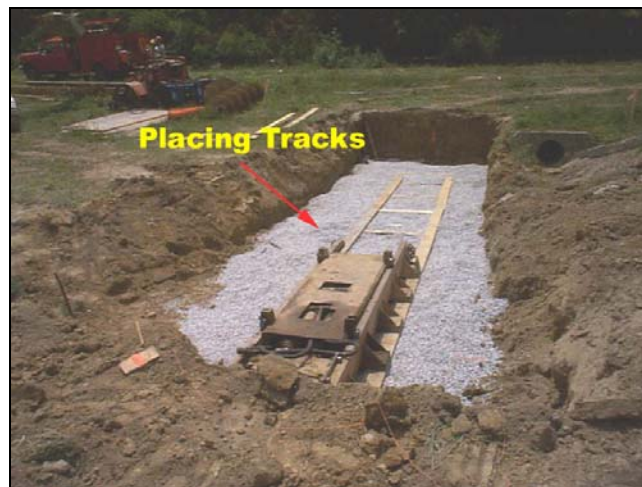
Figure 2.3 Track system for auger boring
