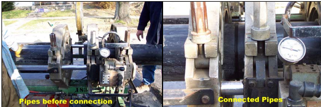
Figure 2.64 Pipe joint using butt fusion
