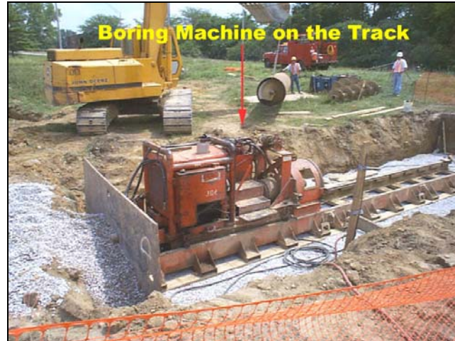
Figure 2.4 Auger boring machine on the track
