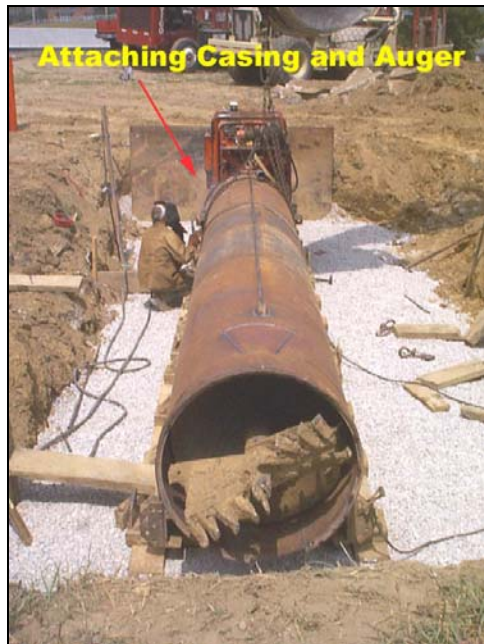
Figure 2.7 Connection of casing and auger
