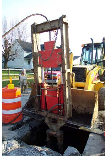
Figure 2.57 Winch for pipe bursting operation
