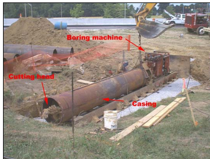
Figure 4.6 Installation of storm water pipe using auger boring
