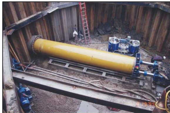
Figure 2.18 Steel casing being jacked (Kerr Construction Inc.)
