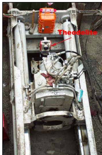
Figure 2.33 Installation of a theodolite
