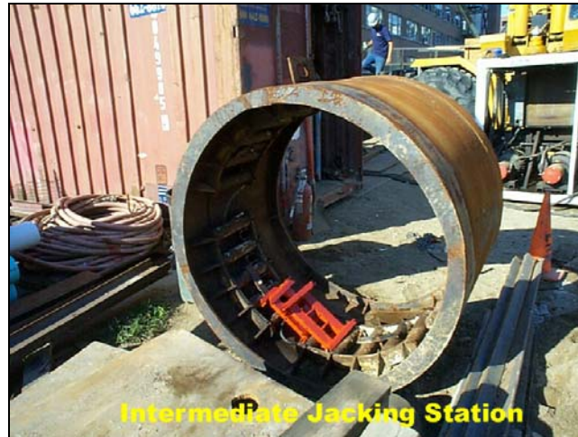
Figure 2.44 Intermediate Jacking Station
