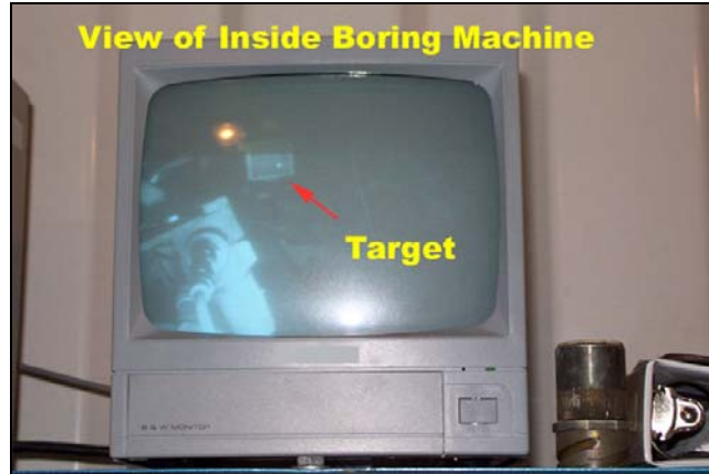
Figure 2.25 Monitor showing a view inside the MTBM
