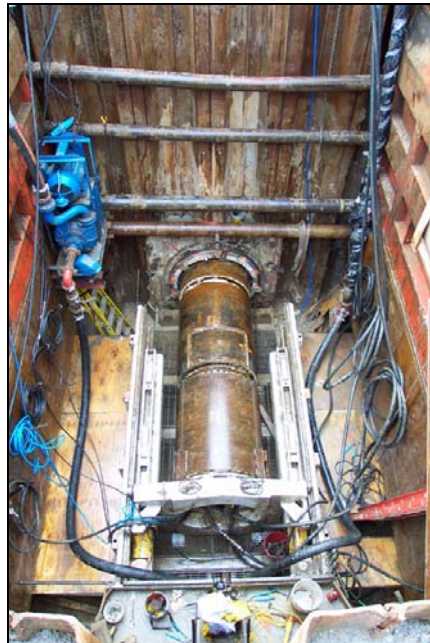
Figure 4.8 Installation of sewer pipe using microtunneling
