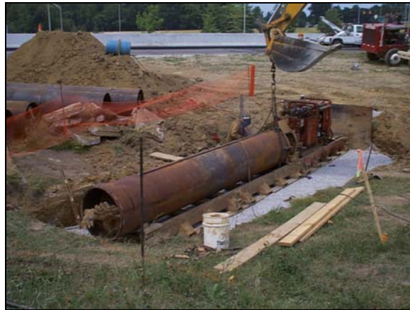
Figure 5.17 Storm water installation using auger boring
