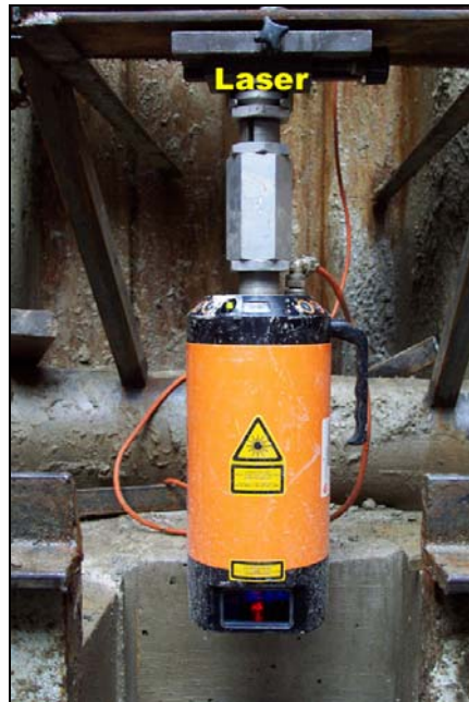
Figure 2.20 Laser for guidance of MTBM
