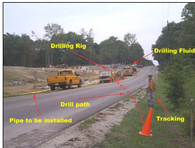
Figure 4.7 Installation of gas line using horizontal directional drilling
