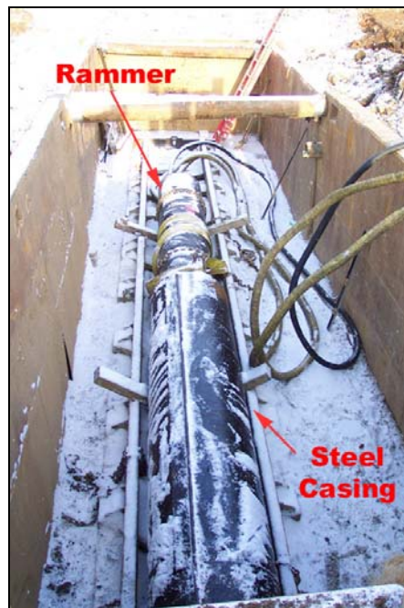
Figure 4.15 Layout of pipe ramming site
