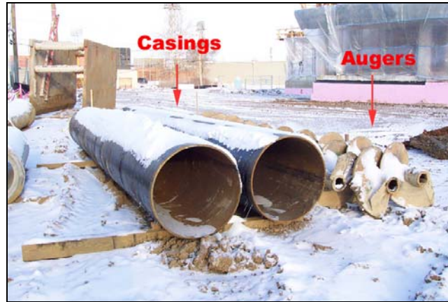
Figure 2.52 Steel casings and augers for pipe ramming projects
