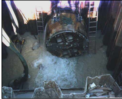
Figure 2.28 MTBM at the receiving shaft (Kerr Construction Inc.)
