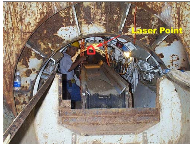
Figure 2.46 Laser point for alignment control
