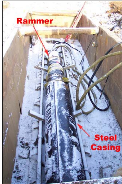
Figure 2.54 Rammer connected to the casing
