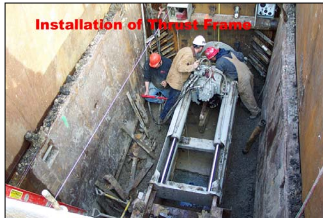
Figure 2.32 Installation of thrust frame
