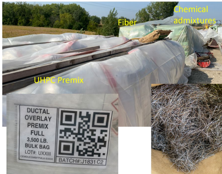
Figure C.3 UHPC materials at the job site.
