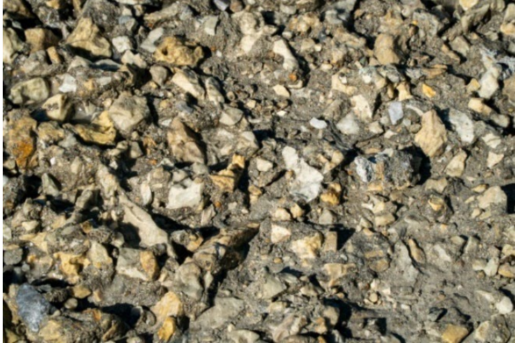
Figure 2.3 Deck surface prepared by hydro-demolition (Haber et al., 2022a).
