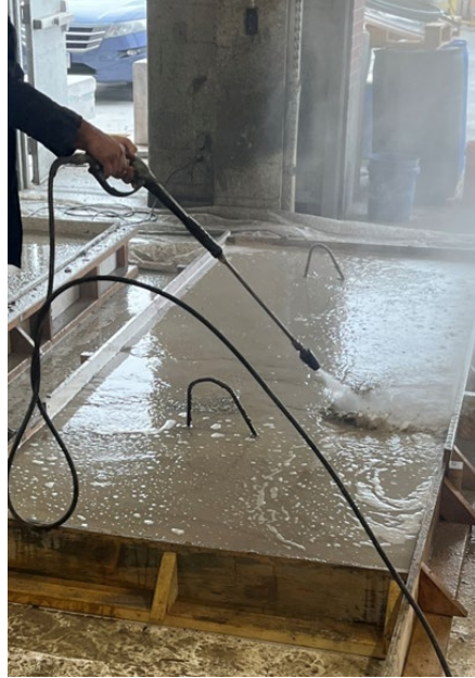
Figure 6.5 Removal of surface retarder using high-pressure water.
