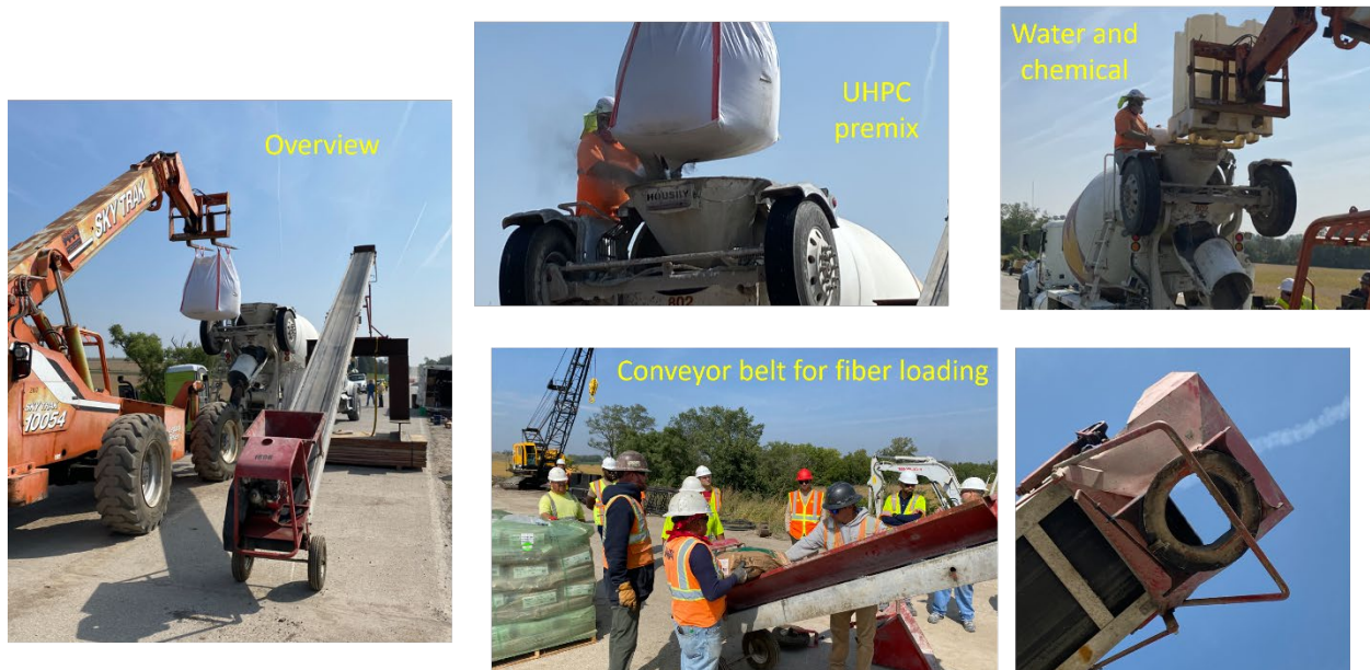
Figure C.4 IADOT Cass County Bridge Overlay Project – Batching.
