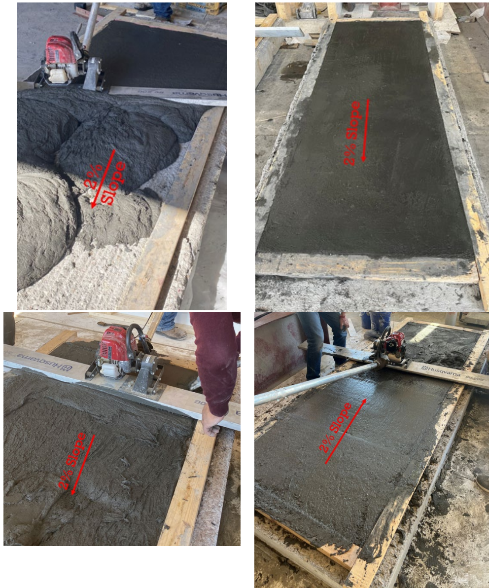
(a) During placement
