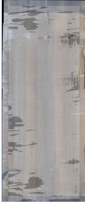
Figure 2.12 Infrared imaging results for Mud Creek Bridge deck (Wibowo et al., 2018).
