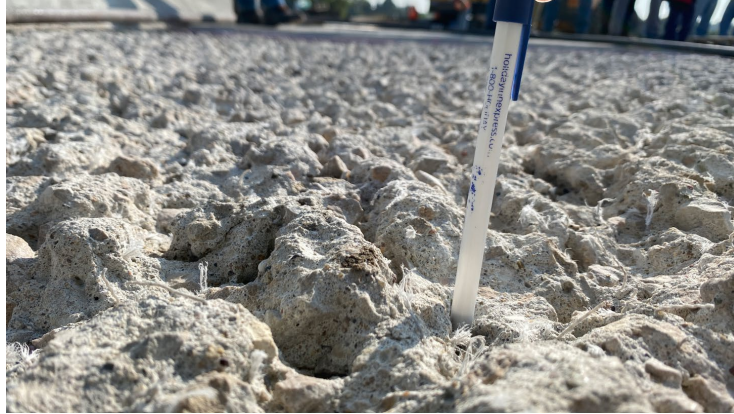
Figure C.1 Surface of bridge deck after hydro-demolition.
