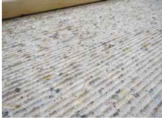
Figure 2.10 Deck surface after grinding (Haber et al., 2018).
