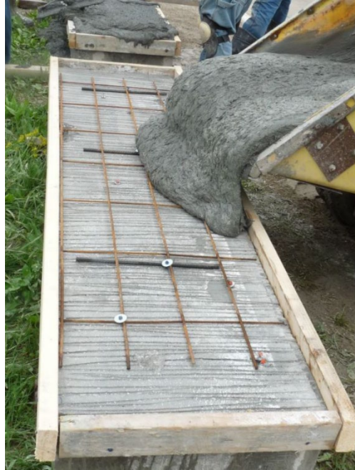
Figure 2.18 Surface preparation on concrete deck used for slab specimens (Wibowo et al., 2018).
