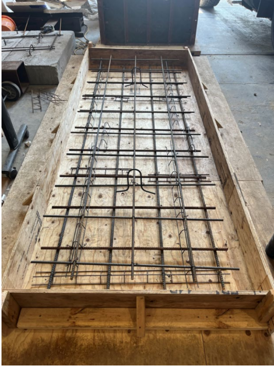
(a) Rebar Placement and Formwork Setup
