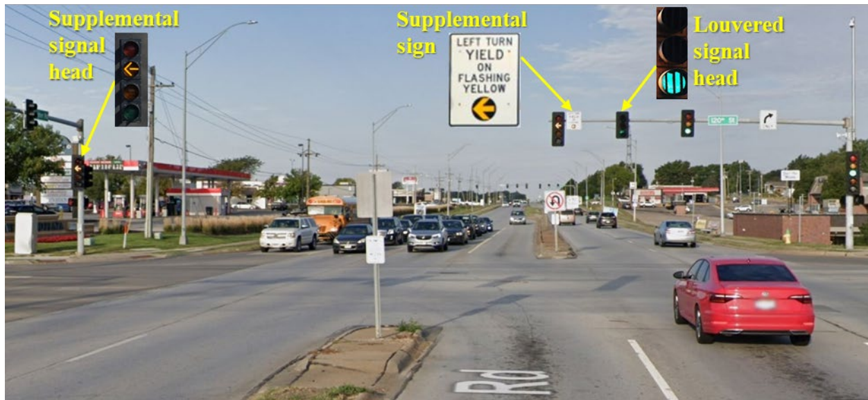
Figure 6.1 Example of the possible treatments implemented at westbound approach of 120th & W Center in Omaha
