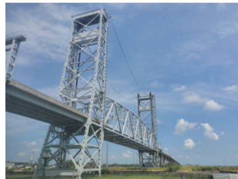
Figure 1. Ellender Ferry Bridge, SR 27, Calcasieu Parish, Louisiana
