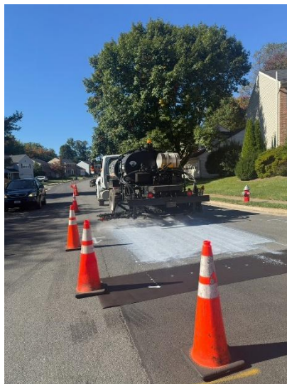
Figure 28. Application of Spray-on Rejuvenator Using an Emulsion Sprayer Truck
