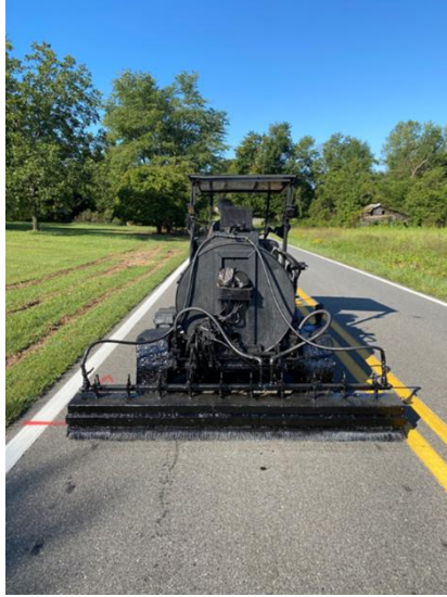
Figure 7. Application of Spray-on Rejuvenator Using a Three-Wheeled Application Unit
