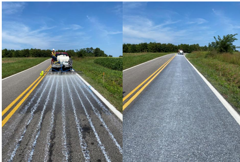
Figure 6. Images of Spray-on Rejuvenator Application Using the Pickup Truck-Mounted Prototype Spray System, Illustrating Initial Non-Uniform Coverage and Subsequent Uniform Application Following Continued Spraying
