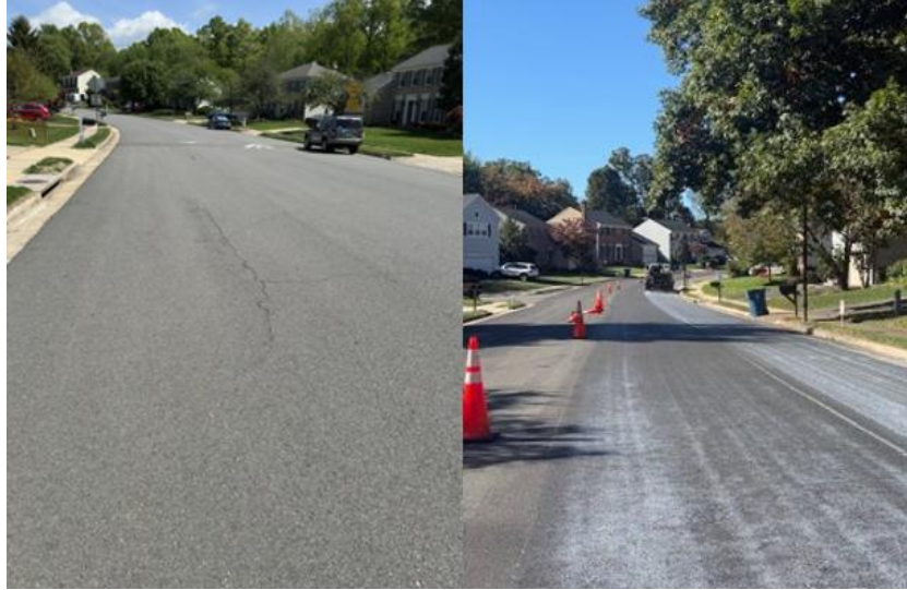
Figure 32. Images of Point Pleasant Drive Before and After Treatment with Product D
