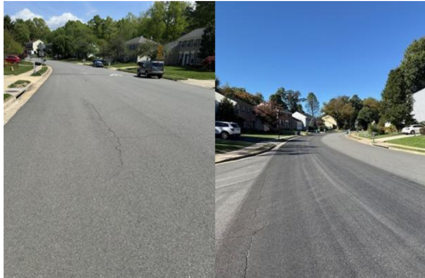
Figure 31. Images of Point Pleasant Drive Before and After Treatment with Product C
