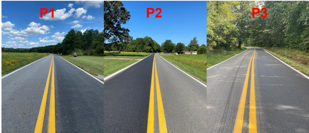
Figure 10. Images of Surface Appearance Shortly after Spray-on Rejuvenator Application for Route 640. P1–P3 denote segments receiving spray-on rejuvenator application.
