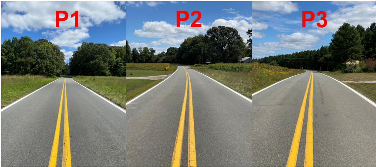
Figure 22. Images of Surface Appearance Approximately 12 Months after Spray-on Rejuvenator Application for Route 640. P1–P3 denote segments receiving spray-on rejuvenator application.
