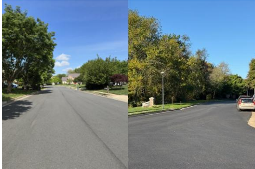
Figure 29. Images of Walney Park Drive Before and After Treatment
