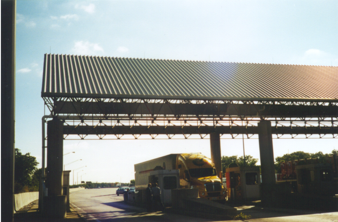
Figure 2.1: Photo of the north end of the Portage Barrier Toll Collection Plaza. View is facing east.
