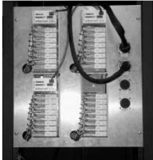
Figure 3-16: Opto22 I/O Modules - Video Detector Status Interpretation (CIVL 21 – CIVL 23)
