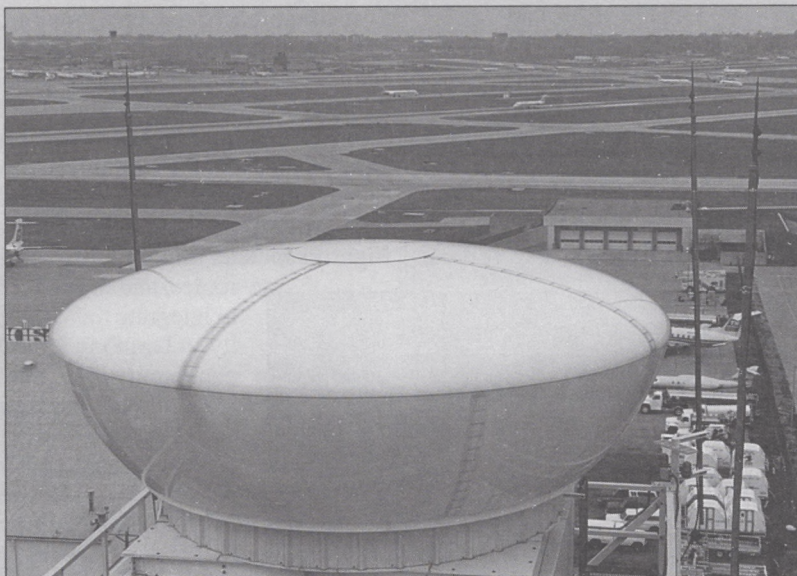
The ASDE-3 antenna (shown here at the St. Louis-Lambert International Airport) monitors ground traffic, enabling air traffic controllers to see positions of aircraft, fuel trucks, and other airport traffic on airport property in all weather conditions.
