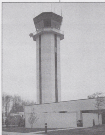
The new airport traffic control tower and terminal radar approach control facility at the Norfolk International Airport in Norfolk, VA.
