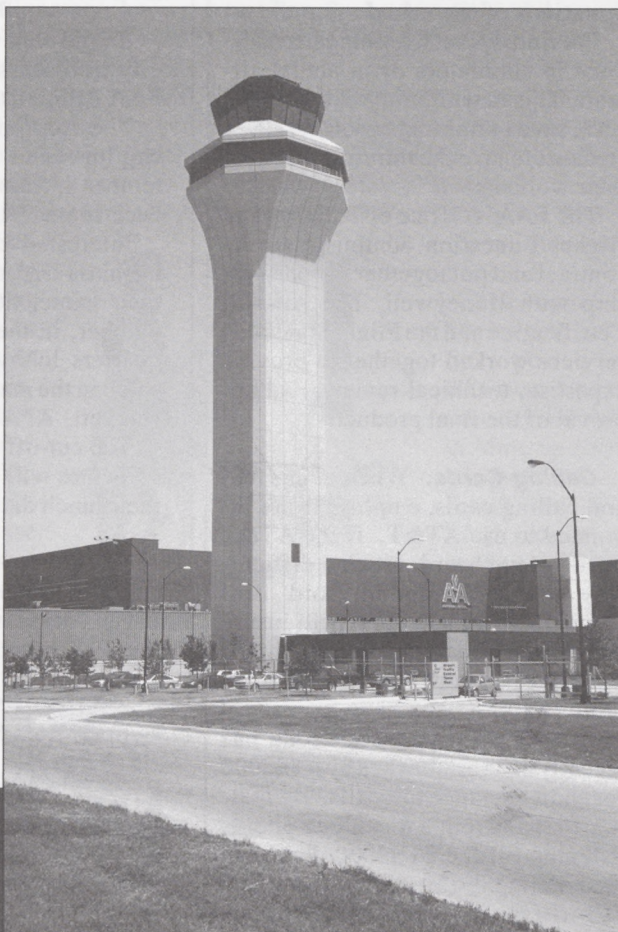
The recently dedicated air traffic control tower on the west side of Dallas/Fort Worth International Airport.
