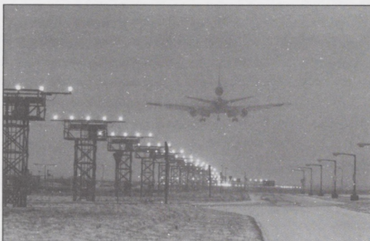
Testing will soon begin at the Technical Center to upgrade the nation's Instrument Landing Systems.
