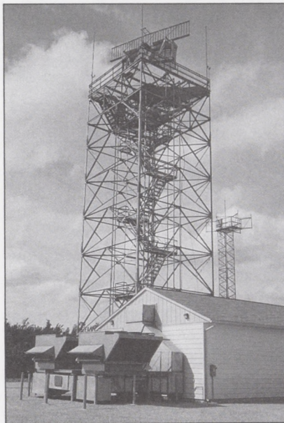
ASR-9 radar equipment in Toledo, OH.
