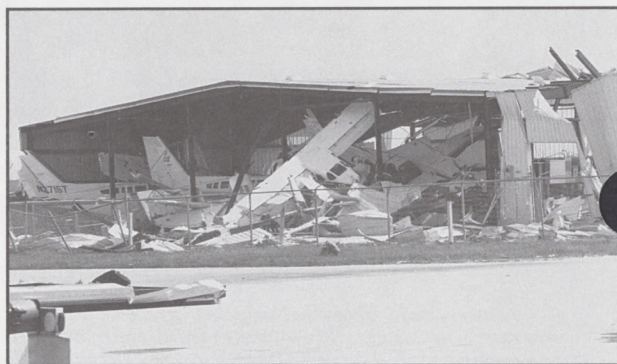
A hangar at the Tamiami airport proved no match for Andrew's fury. The storm's high winds wrecked the facility and the planes it housed.
