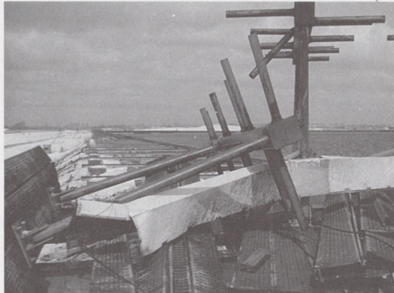
BEFORE: The localizer antenna and counterpoise immediately after the USAir accident.
