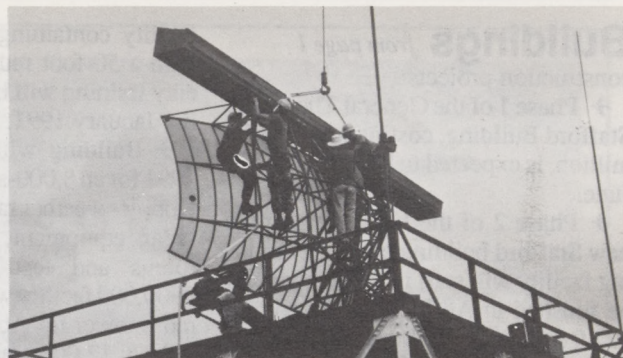
A defective ASR-5 radar antenna is replaced on Panama's Perico Island.
