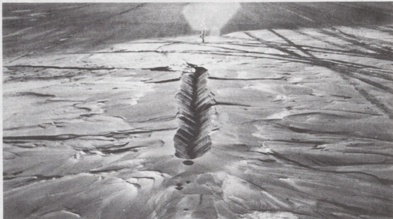
The surface beneath Oakland International Airport is composed of loose sandy soil. Beneath the soil is water. During the earthquake, the tremors caused the water to rise, mix with the soil and liquify the soil. This mixture came through cracks on the runway surface.
