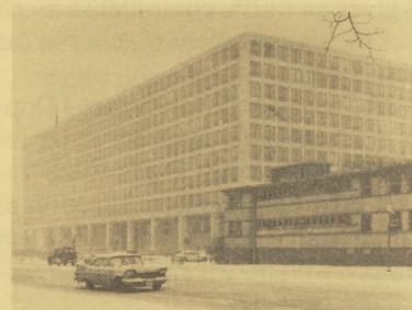
A month after the new building opened, snow blankets Independence Avenue and a finned automobile. To the right was an old building used by the Navy.
