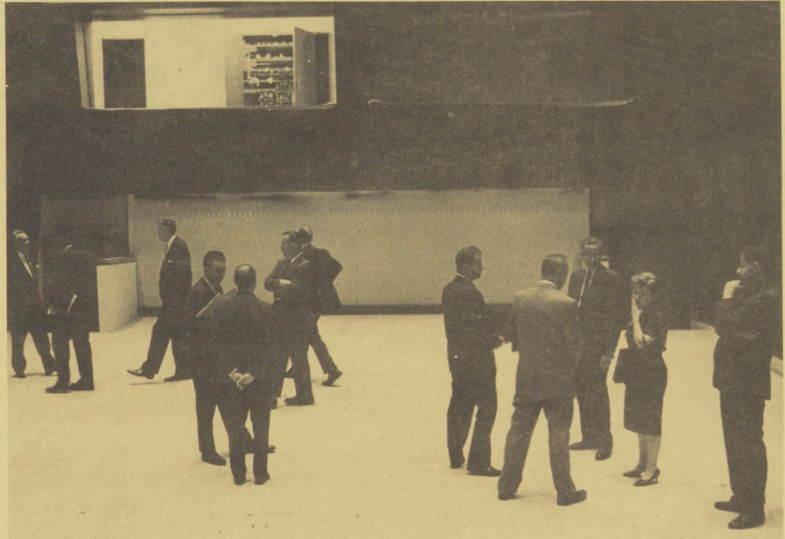
The task force inspects construction of FAA's third-floor auditorium. Mary Healy, second from right, recalls the group's long hours of work to get the building ready in the fall of 1963.
