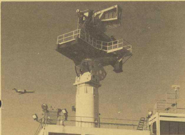
The new ASR-9 antenna will soon be seen at radar sites around the country.
