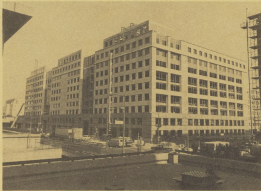
The new Aerospace Center building on D Street is expected to be ready for occupancy this fall.
