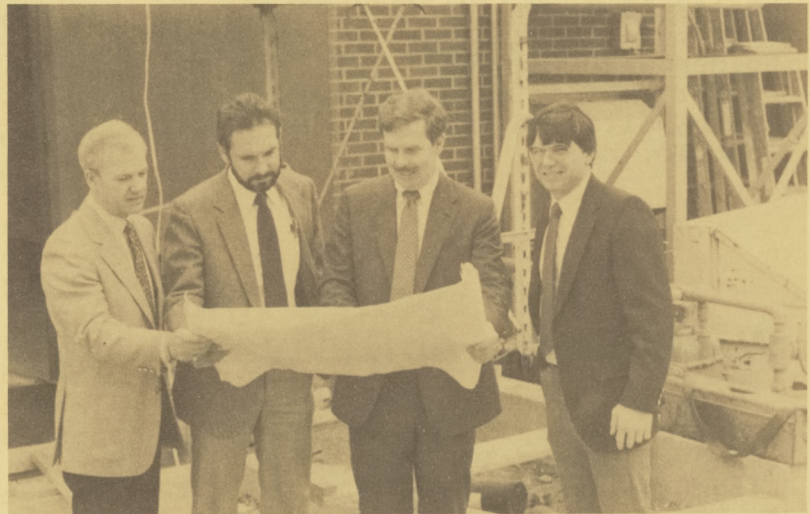
Studying plans for a $555,000 modernization of the Greater Cincinnati International Airport are Covington, KY, AFS members, (L to R) David Bullock, Manager; William Stevie and Karl Weisenberger, both supervisors; and Wayne Rogers, Assistant Manager
