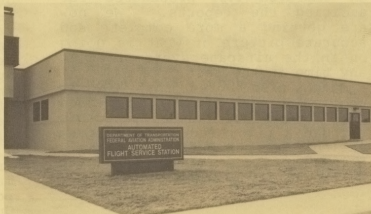
The Washington Automated Flight Service Station, located in Leesburg, Va., was commissioned in late August and is now fully operational.
