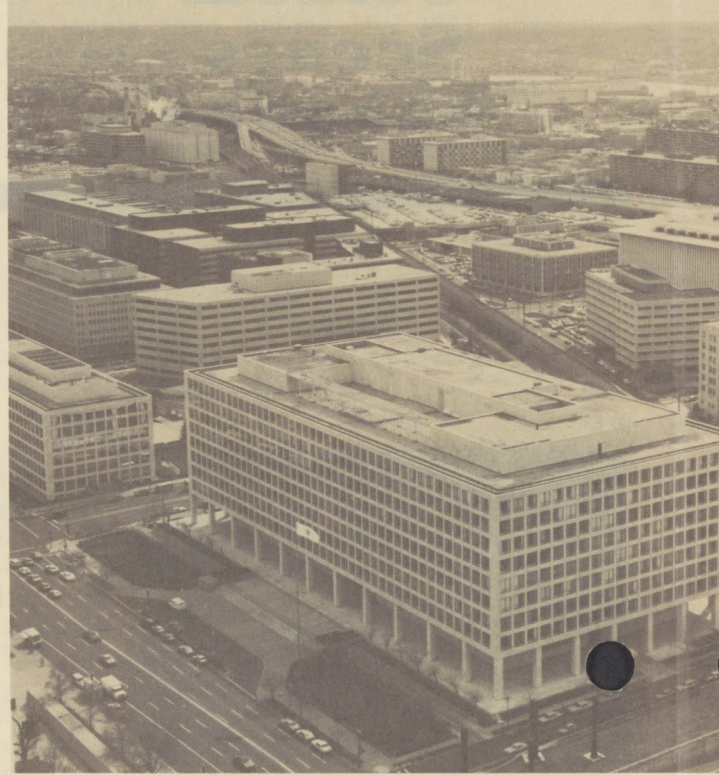
The now defunct heliport atop FOB-10A is barely discernable in this view.
