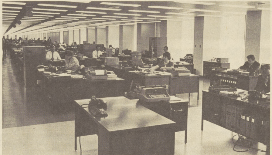
Before partitions became popular, some "bays" extended the entire length of the building.
