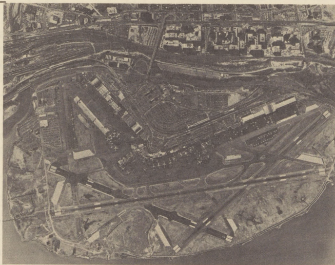
During a major safety modification project, overrun areas at Washington National Airport are being extended. See 4.
