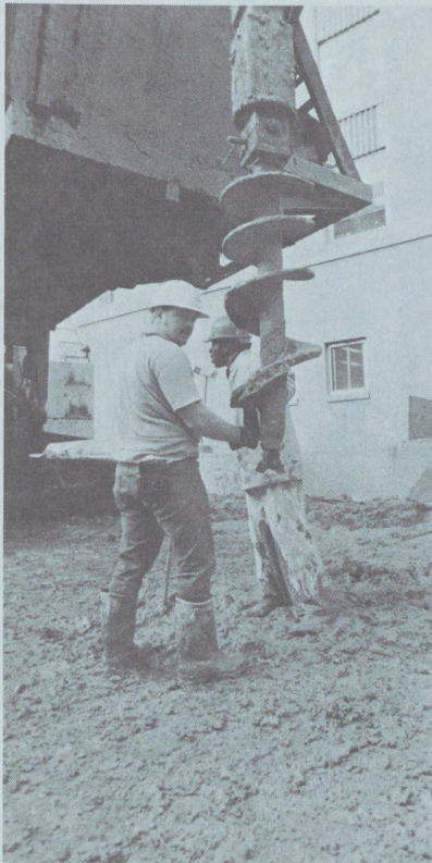
Giant bit cuts into hard earth under the mud.
