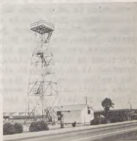
SURVEILLANCE RADAR TOWER
