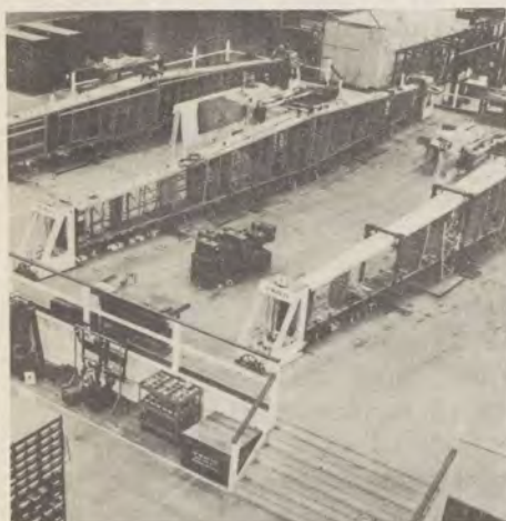
ASSEMBLY OF MAIN WING SPARS
