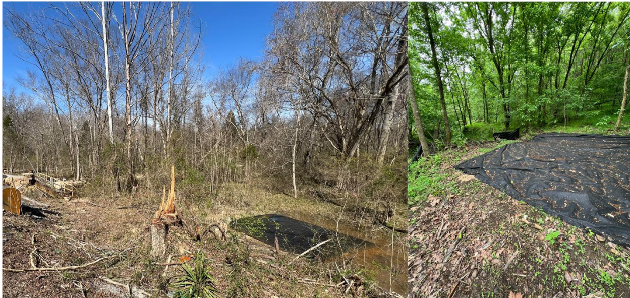
Figure 4. Dewatering Operations at Site 1 (left) and Site 2 (right)
