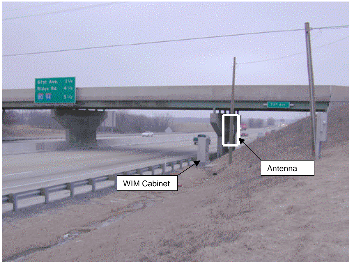
Figure 4-5: Antenna at WIM Station 4410 on I-65 Northbound at Milepost 253.62
