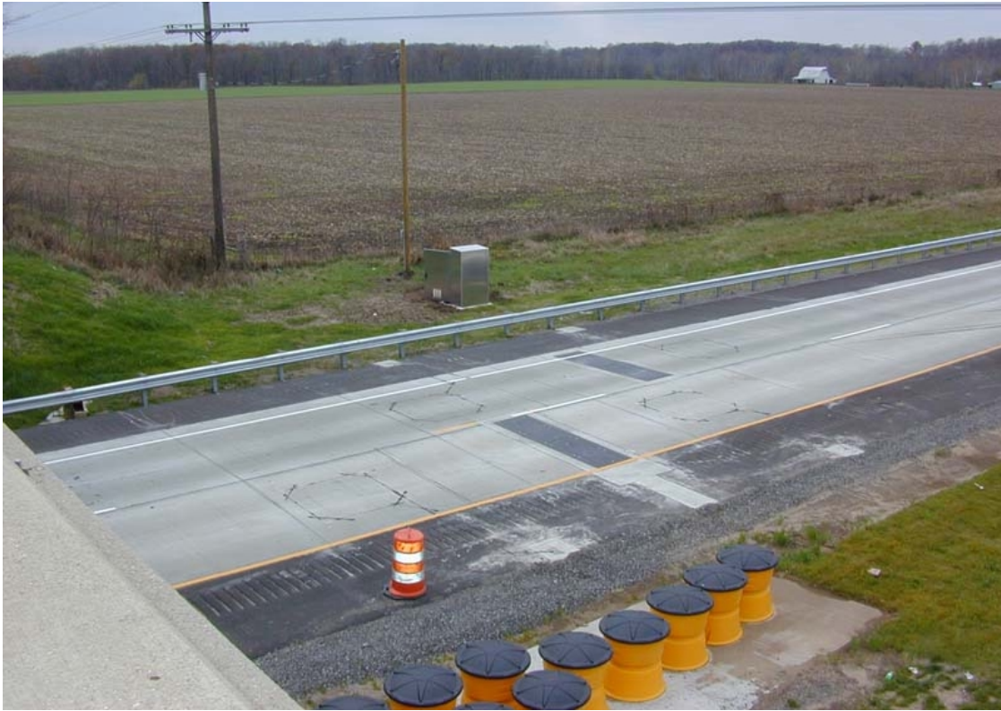
Figure 3-5: Single load cells in each lane, I-74 WB, near Covington, IN
