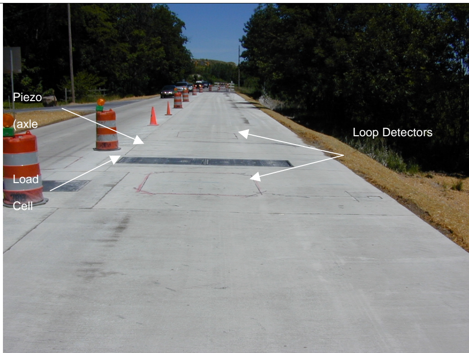
Figure 2: WIM scales (during construction ~July 2001).
