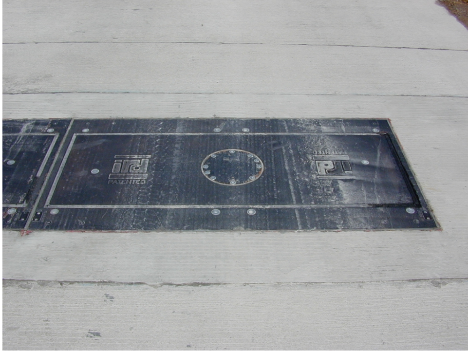
Figure 3: WIM load cell.
