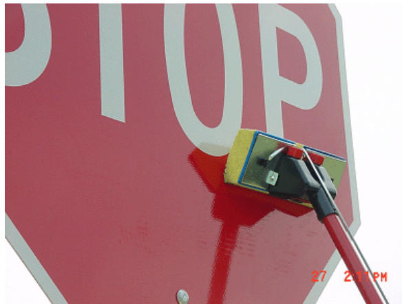
Figure 3-7: Picture of Dry Mop used to Wipe Signs
