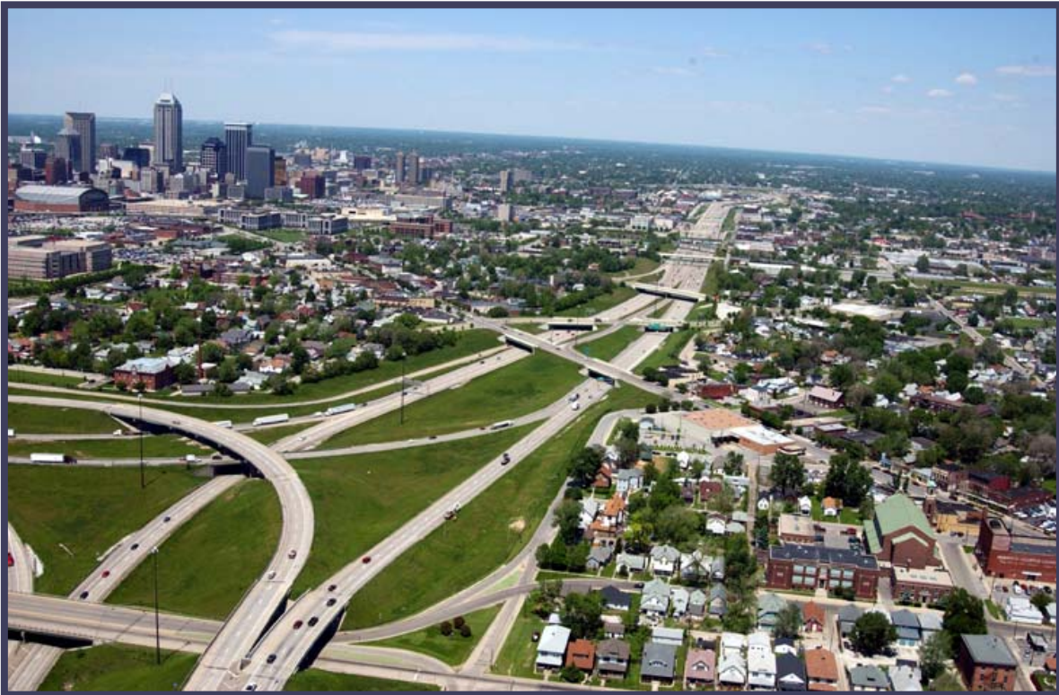
Figure 3 – South Split Looking North
