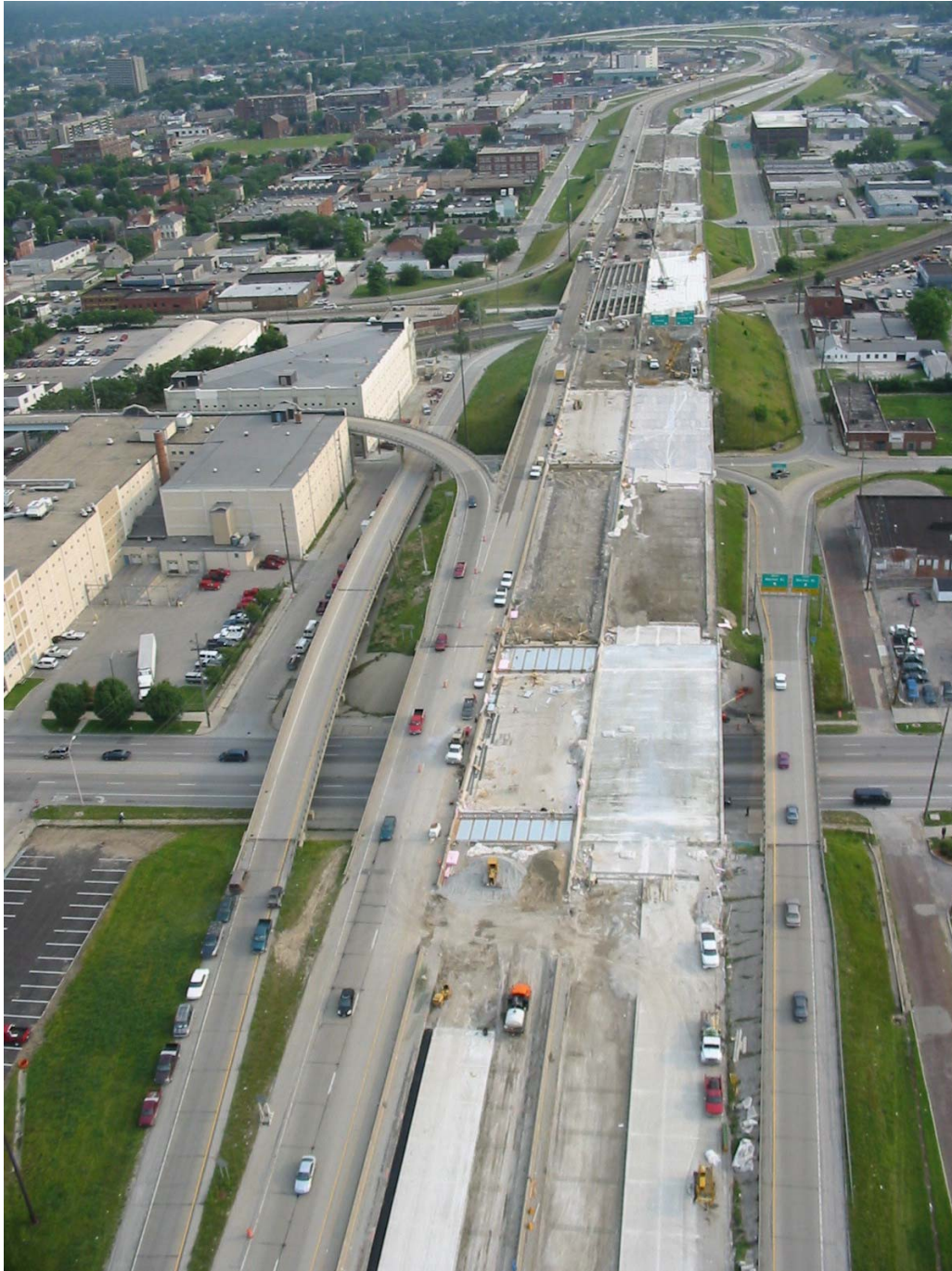
Figure 4 – Main Line During Closure Looking North
