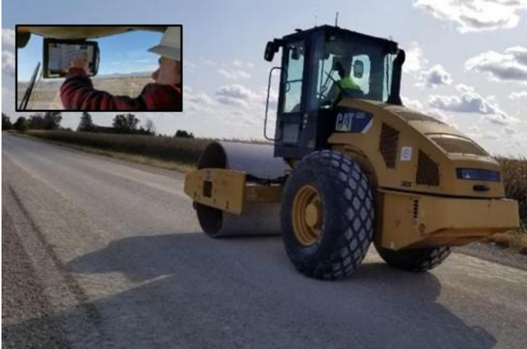
Figure 1. COMP-Score® RT enabled roller performing modulus mapping on an unpaved roadway
