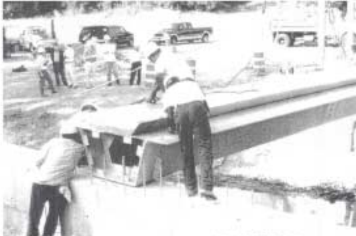
Figure 3.13. FRP support beam (Foster et al. 2000)
