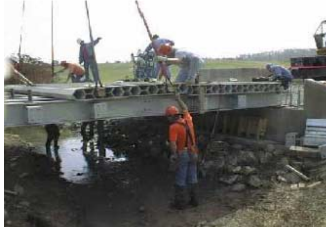
Figure 3.20. Superdeck bridge deck panels
