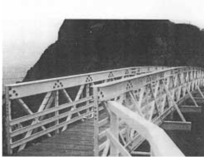
Figure 3.1. 70-ft long FRP pedestrian bridge (Johansen et al. 1997)
