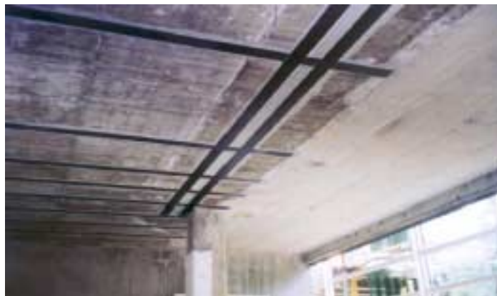
Figure 2.10. Atlas carbon laminates installed on underside of a concrete slab
