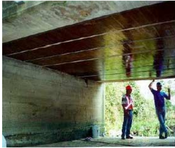
Figure 2.12. MoDOT Bridge G270 (Iron County, MO)
