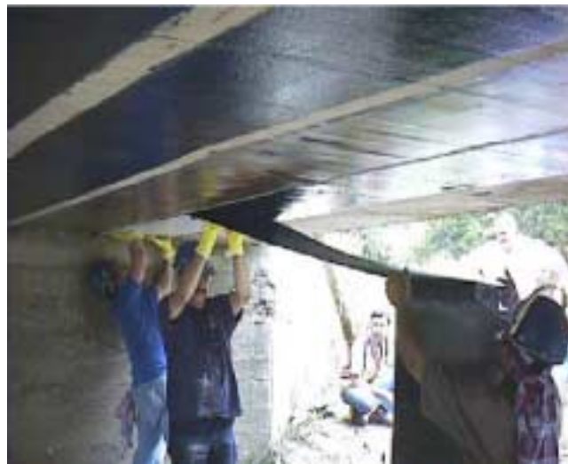
Figure 2.9. Installation of the CFRP sheets (Mayo et al., 2000)
