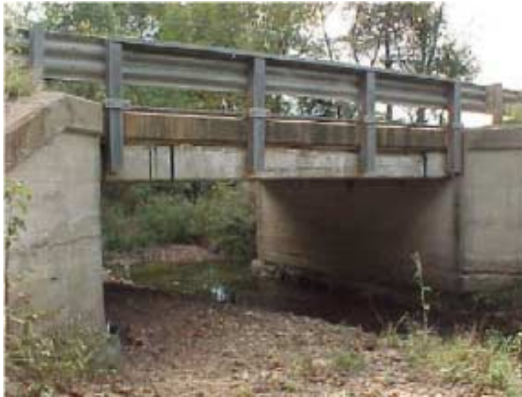
Figure 2.7. Bridge G-270, Missouri (Mayo et al., 2000)
