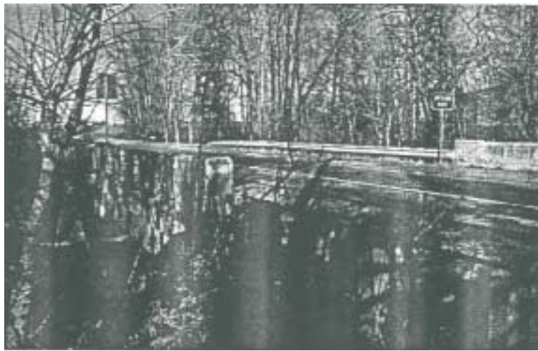
Figure 3.4. Bridge 1-351 (Chajes, M. et al. 1998)
