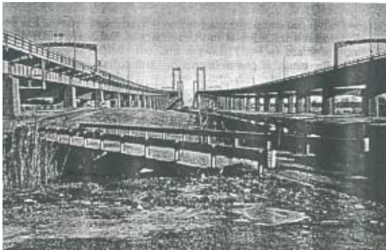
Figure 3.3. The Magazine Ditch Bridge (Chajes, M. et al. 1998)
