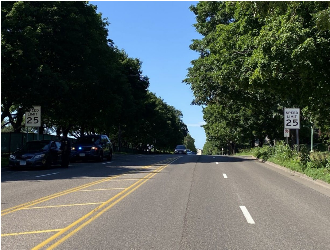
Figure 21. Oversized speed limit signs on both sides of the road greet drivers on Cretin Boulevard heading north
