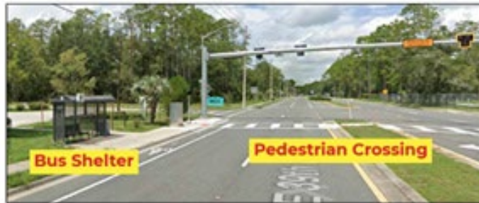
Figure 11. Upgraded bus stop, ADA accessibility, and pedestrian hybrid beacon on NE 39th Avenue (Source: City of Gainesville)
