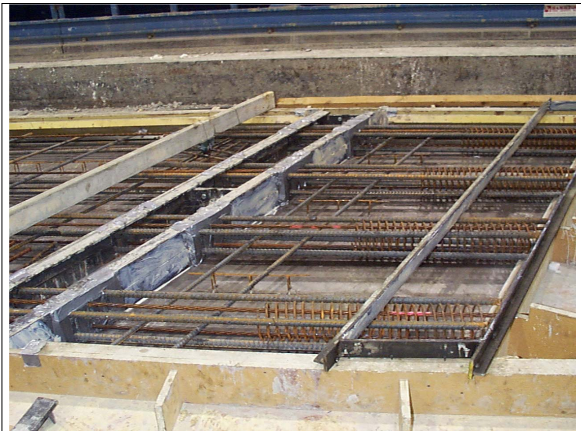
Fig. 62. Spiral confinement at panel overhang (JDV, 2003)
