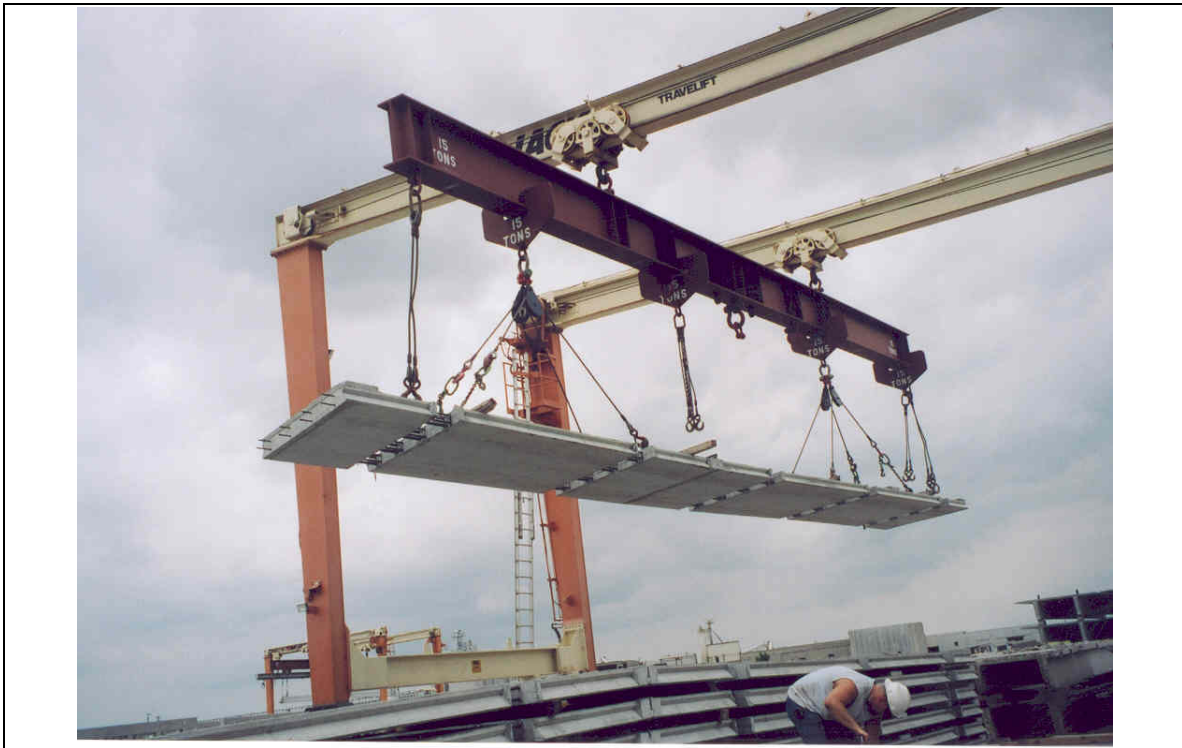
Fig. 73. Typical NU-Deck panel lifted with eight anchor devices before setting (Versace, 2003)
