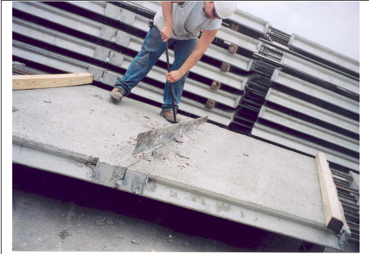
Fig. 74. Removal of plate at hinge section to form the panel crown (Versace, 2003)
