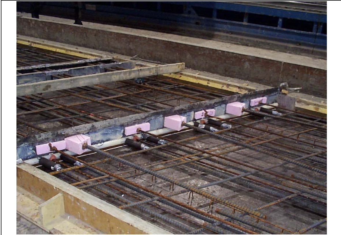
Fig. 72. Typical NU-Deck panel hinge section ready for concrete (Versace, 2003)
