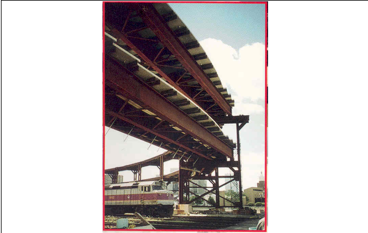
Fig. 121. Transverse Inverset Bridge System units (The Fort Miller Co., Inc., 1998)
