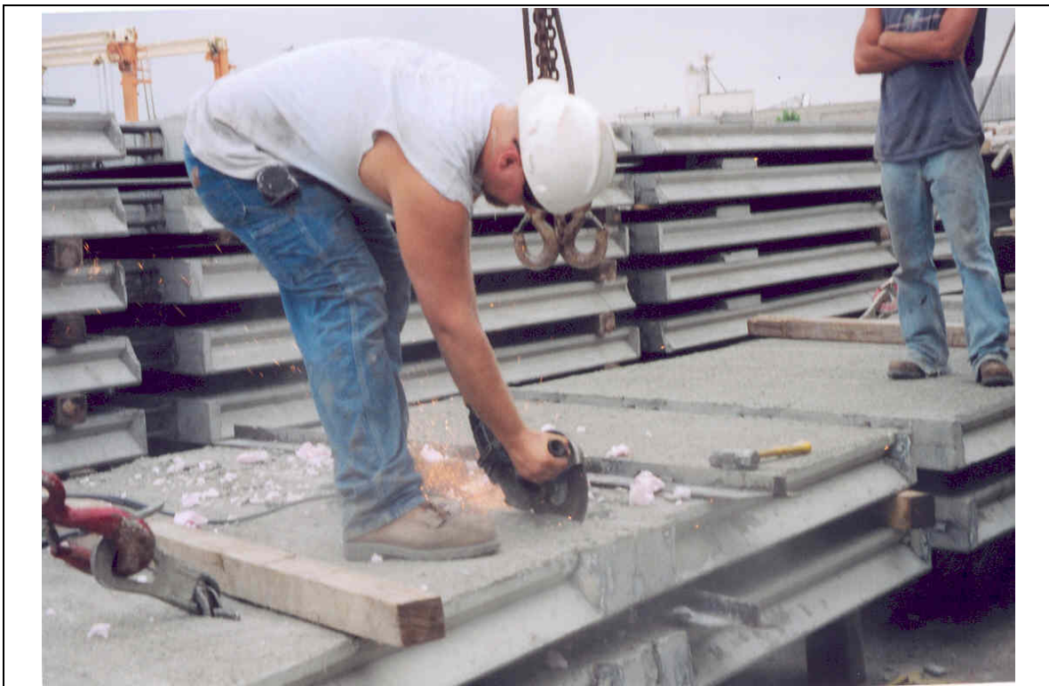
Fig. 75. Cutting of top strands at hinge section to form the panel crown (Versace, 2003)
