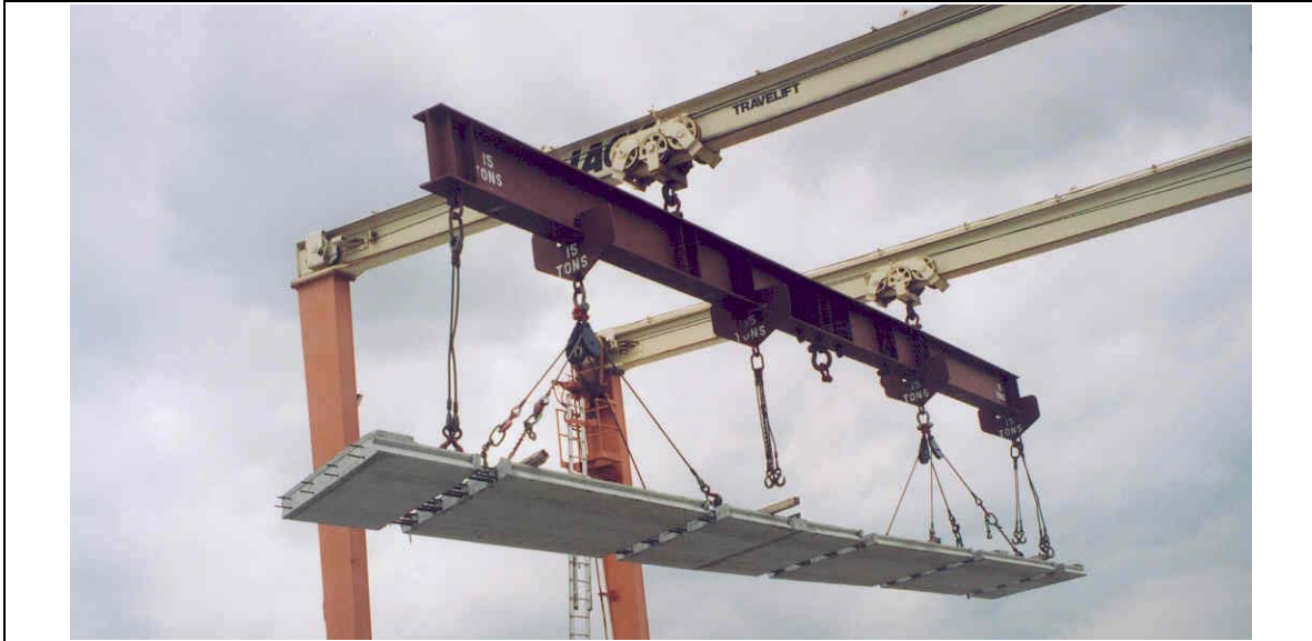
Fig. 3. Typical NU-Deck panel for a bridge in Omaha, NE (JDV, 2003)
