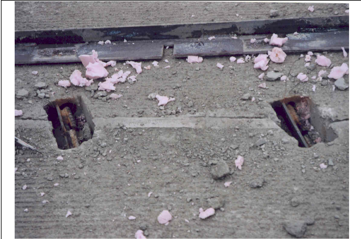
Fig. 76. Plates welded to reinforcing bars at hinge final position (Versace, 2003)
