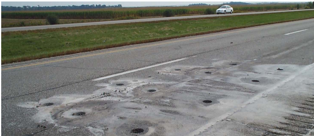
Figure 20: Coring locations in the pavement, Site 1.
