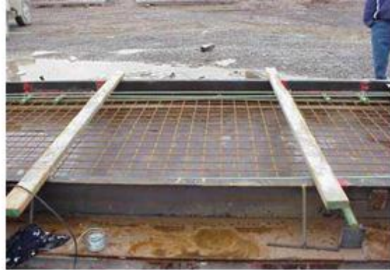
[b] Reinforced Bars
