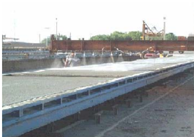
Figure 4.17 Double-coat of curing compound was applied
