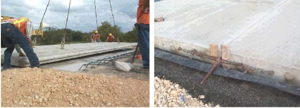
Figure 4.26 Place the base panel next to the joint panel and tie two panels together
