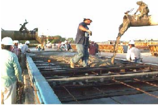
Figure 4.14. Filling concrete in forms of panels
