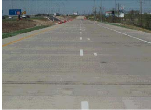
Figure 4.38 The finished precast pavement project in Georgetown, Texas
