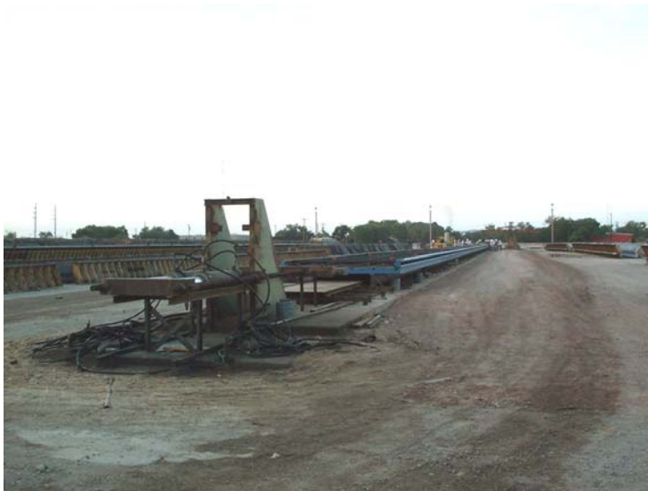
Figure4.7. The Precast Prestressed Concrete Panels Fabrication plant
