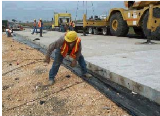
Figure 4.35 The strands will be threaded through the ducts in the panels
