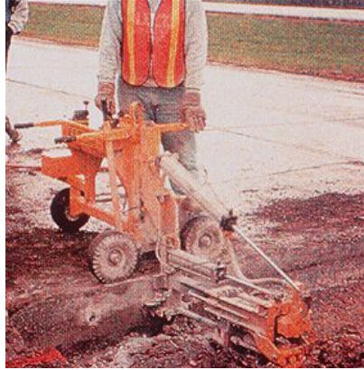
Figure 8.5 Drilling Dowel Slots (26)
