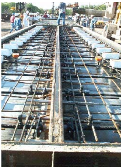
Figure 4.12. Small boxes/inserts are placed in for preparing access pockets of joint panel mold
