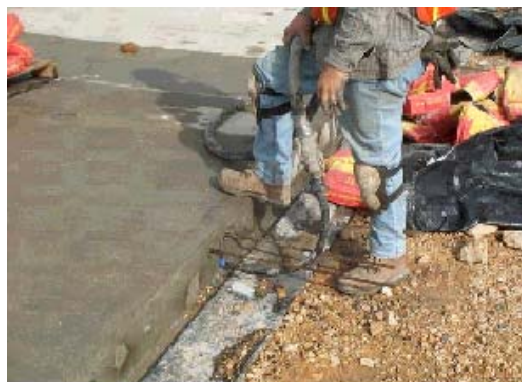
Figure 4.37 Grouting
