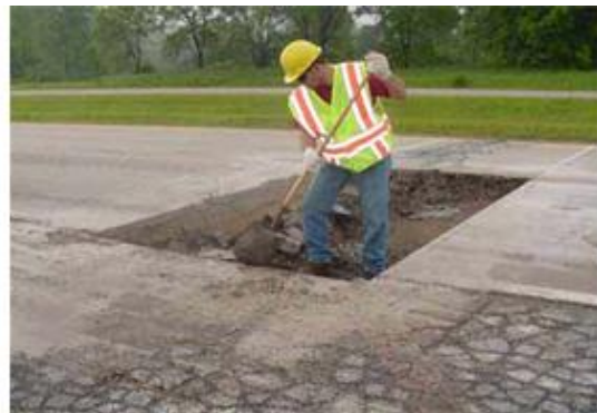
Figure 7.3 Base Preparation (24)
