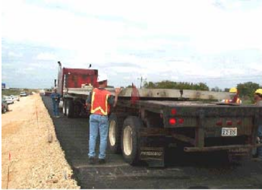
Figure 4.22 Transport panels to worksite
