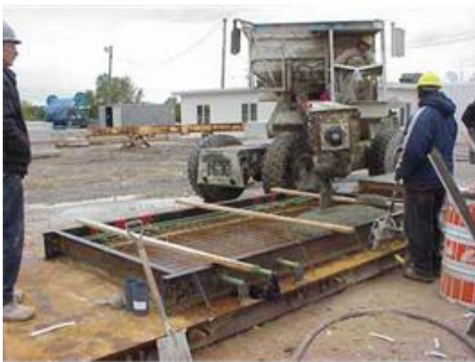
[c] Pouring Concrete
