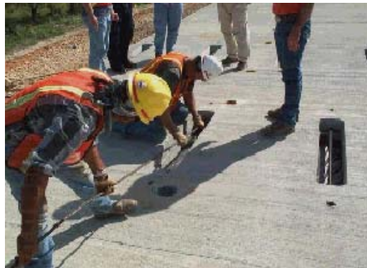
Figure 4.29 Strands will be threaded through the stressing pockets from the central panels
