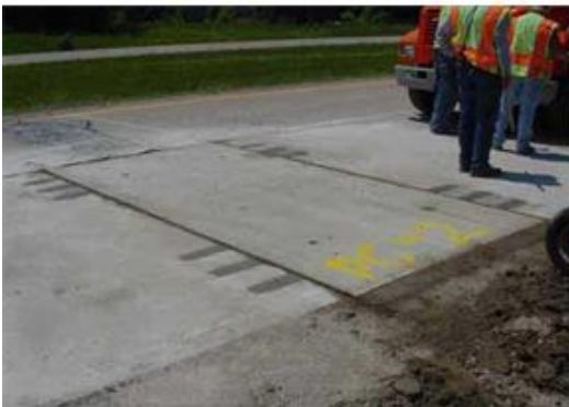
Figure 7.6 Precast Panel Installation (24)
