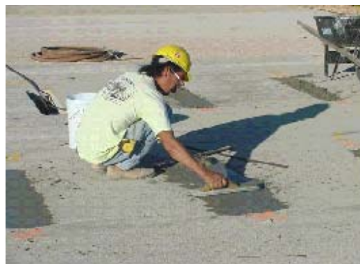
Figure 4.32 Finish the stressing pockets with fast-setting concrete
