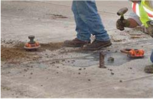
Figure 7.2 Lift Hook Installation and Slab Removal (24)
