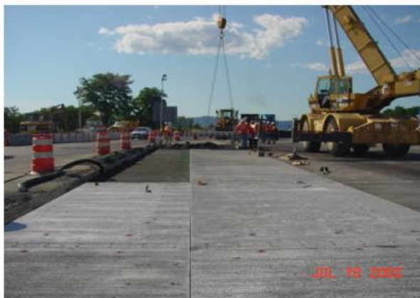
Figure 5.4. Super-Slab Installation (18)
