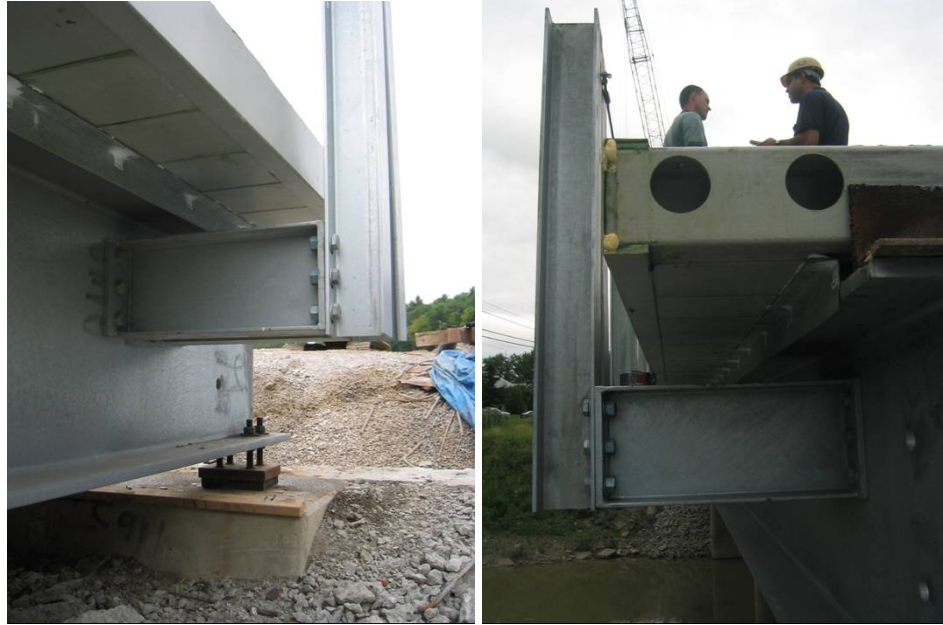
Figure 4-16 Guardrail cantilevered from girders
