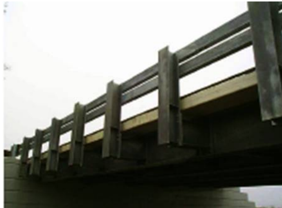
Figure 2-15 Steel Guardrail Cantilevered from Girders (Source: MMC 2003)
