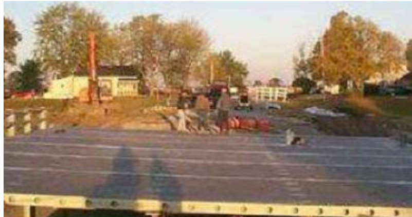
Figure 5-13 Finish panel installation (Source: Busel and Lockwood 2000)
