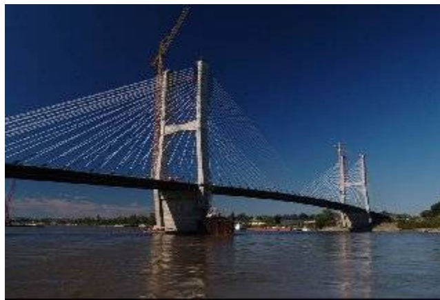
Figure 5- 17 Cape Girardeau Bridge, Cape Girardeau, Missouri
