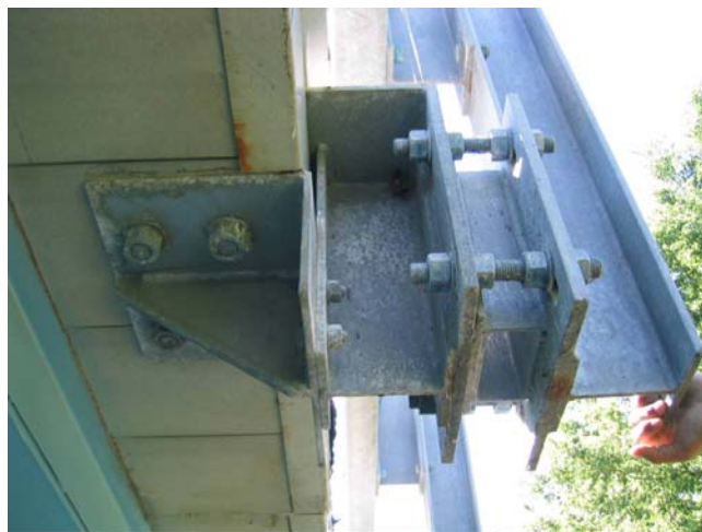
Figure 4-18 Guardrail attached to deck
