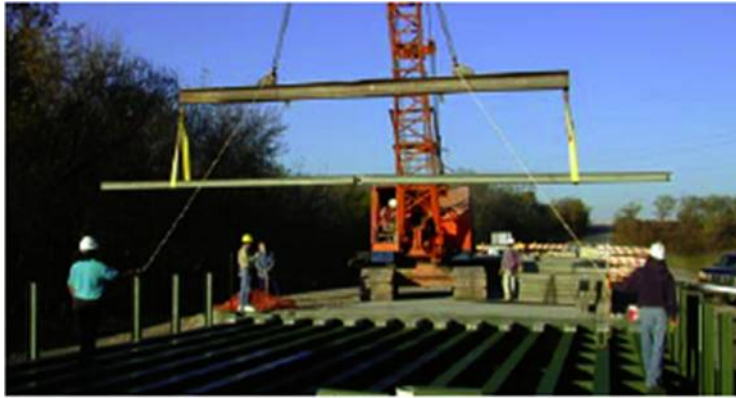
Figure 2-19 Installation of the KSCI's FRP Composite Deck (Source: KSCI 2003)
