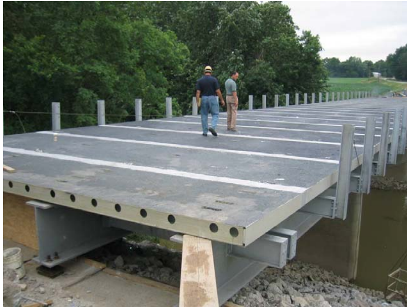
Figure 4-14 County line road over Tiffin River
