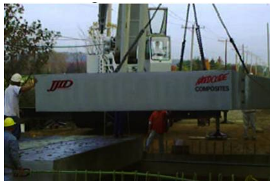
Figure 2-11 Installation of 32 ft. x 13 ft. Longitudinal Panels on Abutments (Source: Hardcore 2003)
