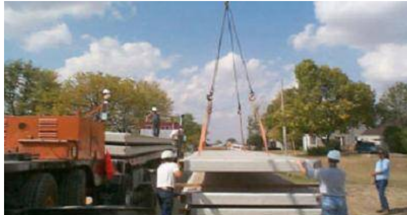
Figure 5-5 Panels being unloaded (Source: Busel and Lockwood 2000)
