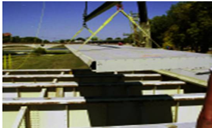
Figure 2-16 Lifting Deck Panel Using Nylon Strap (Source: CPI 2003)
