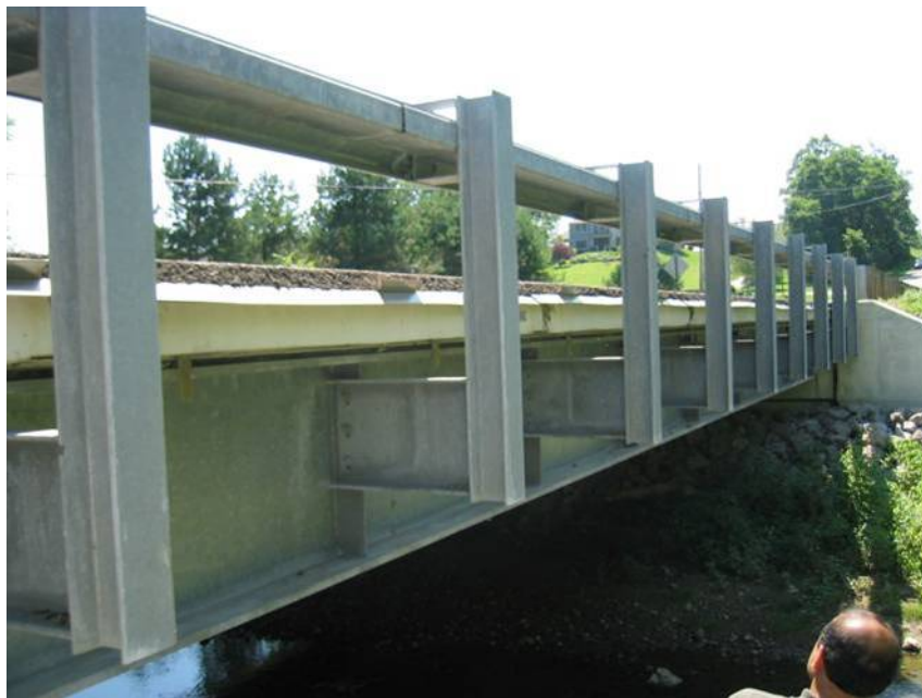
Figure 4-12 Guardrail cantilevered from girders
