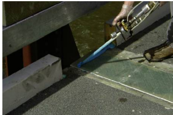
Figure 2-12 Installation of Splice Plates and Bonded FRP Curbs (Source: Hardcore 2003)
