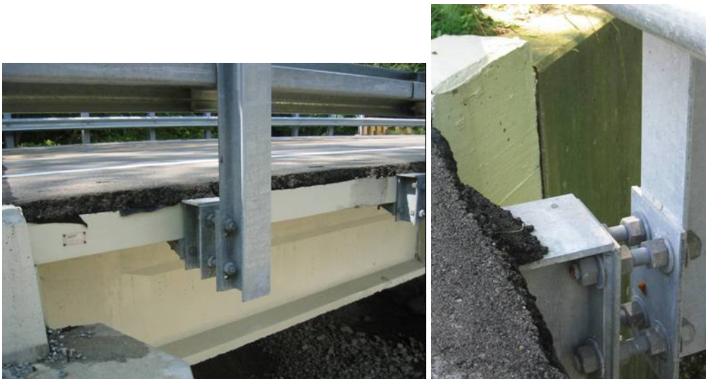
Figure 4- 24 Guardrail attached to deck
