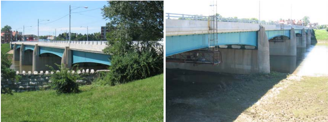
Figure 4-3 Salem Avenue Bridge
