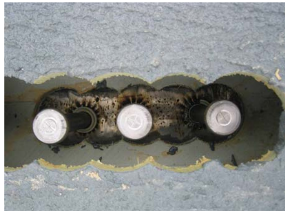
Figure 5-14 Connect decks with girders
