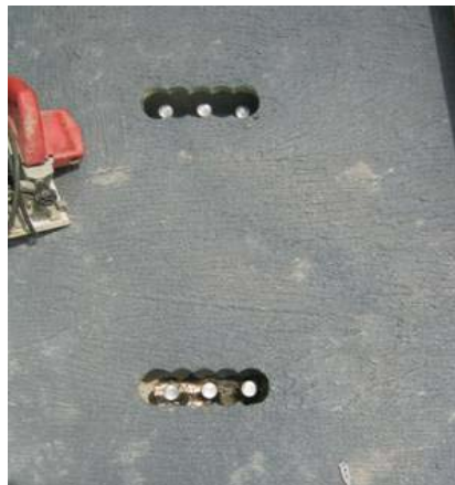
Figure 5-14 Connect decks with girders
