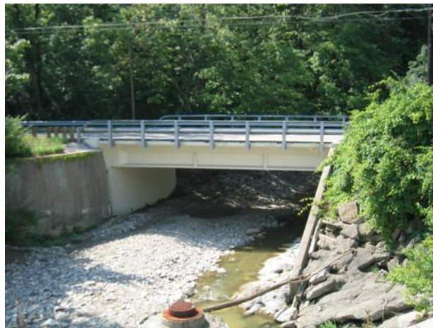
Figure 4-21 Five Mile Road Bridge # 0171
