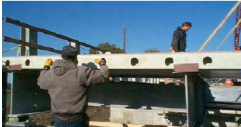
Figure 5-7 Install and align first panel (Source: Busel and Lockwood 2000)
