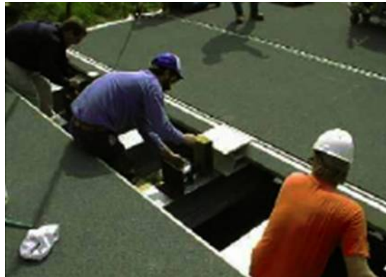
Figure 2-18 Joining Panels Together with Hydraulic Jacks (Source: CPI 2003)
