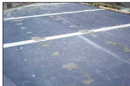
(e) After non-shrink grouting
