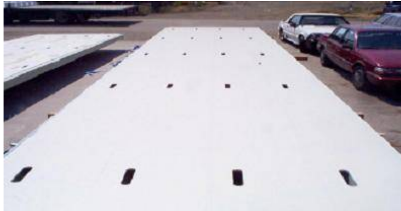
Figure 5-3 Panels finished for loading (Source: Busel and Lockwood 2000)
