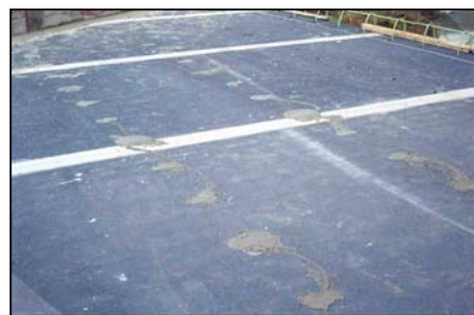
(e) After non-shrink grouting
