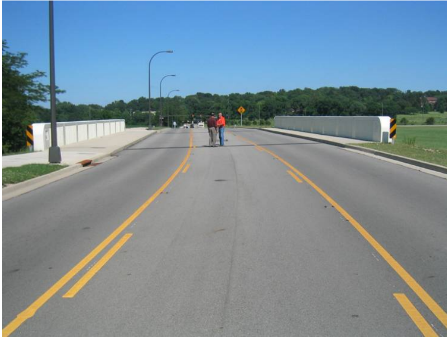
Figure 4-7 Westbrook Road Bridge over Dry Run Creek
