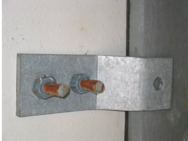
Figure 4-9 Steel S-Clip attached to studs along bottom of panels
