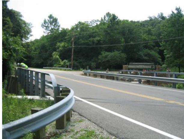
Figure 4-22 Five Mile Road Bridge #0087
