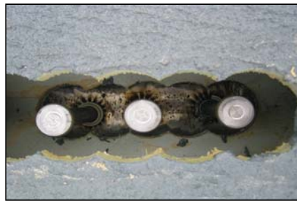
(b) After welding shear studs
