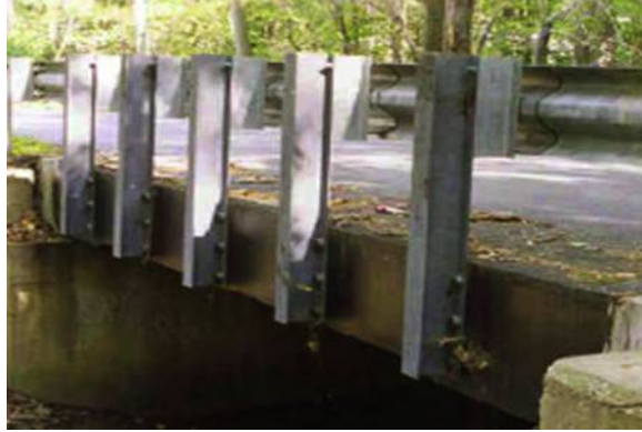
Figure 2-13 Side-Mounted Guardrail on Vehicle Bridge (Source: Hardcore 2003)
