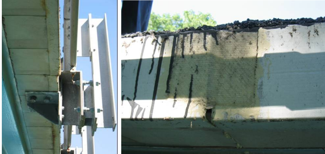
Figure 4- 20 Keeping tolerance around deck edge with guardrail straight
