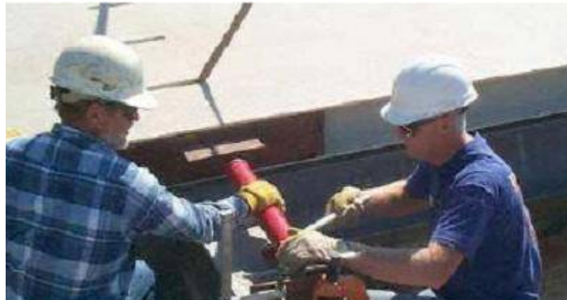
Figure 5-11 Align the panel using a jack (Source: Busel and Lockwood 2000)
