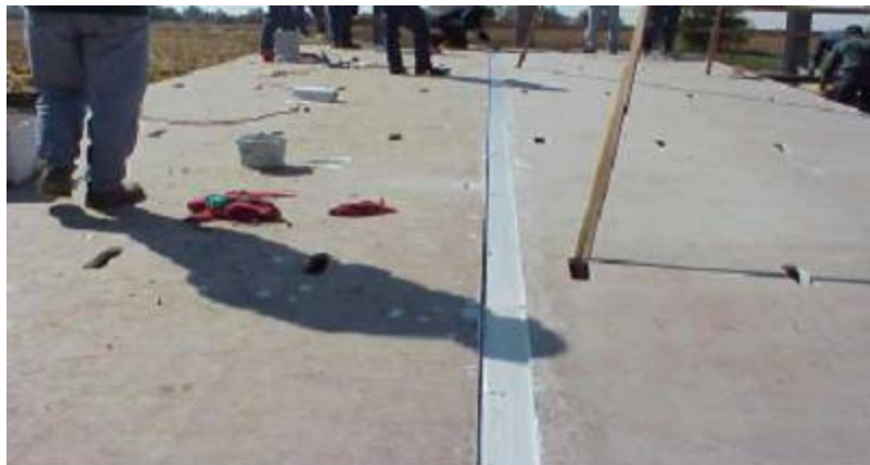
Figure 5-10 Lowering of second panel (Source: Busel and Lockwood 2000)
