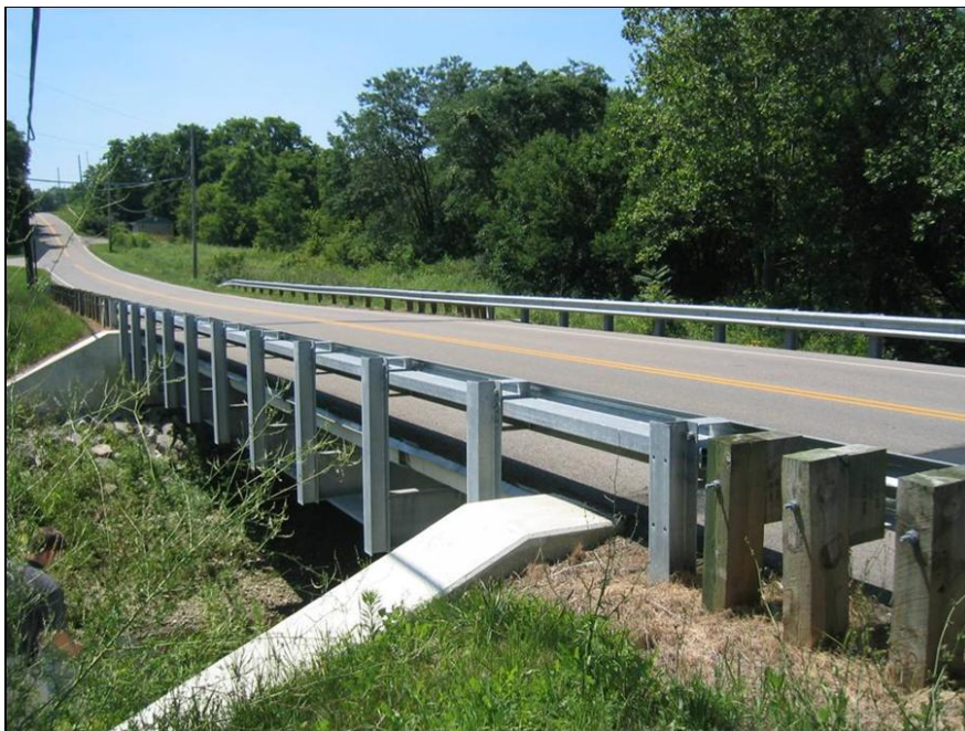
Figure 4-8 Sintz Road over Rock Run Bridge
