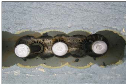
(b) After welding shear studs
