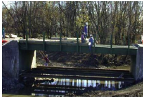
Figure 2-20 Bolting Down FRP Composite Deck (Source: KSCI 2003)
