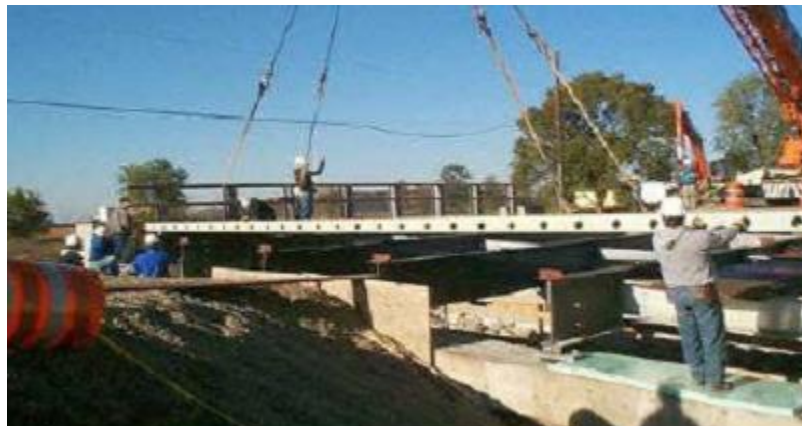
Figure 5-6 Install first panels (Source: Busel and Lockwood 2000)
