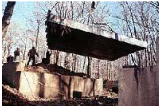
Figure 2-9 Installation of a Single 20 ft. x 26 ft. Bridge Panel (Source: Hardcore 2003)
