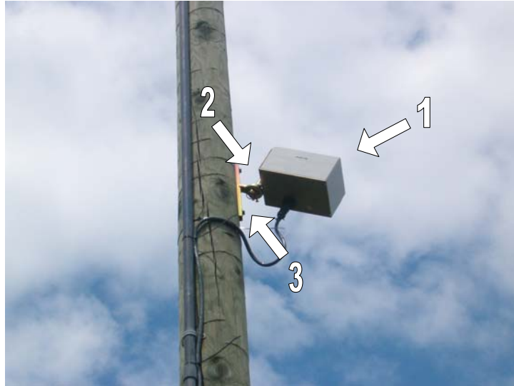
a) Radar Traffic Microwave Sensor (RTMS)
