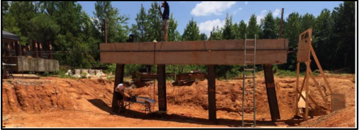
Figure 2-1 Multi-span bridge with cast-in-place reinforced concrete bents supported on H-piles (Anderson et al., 2018)
