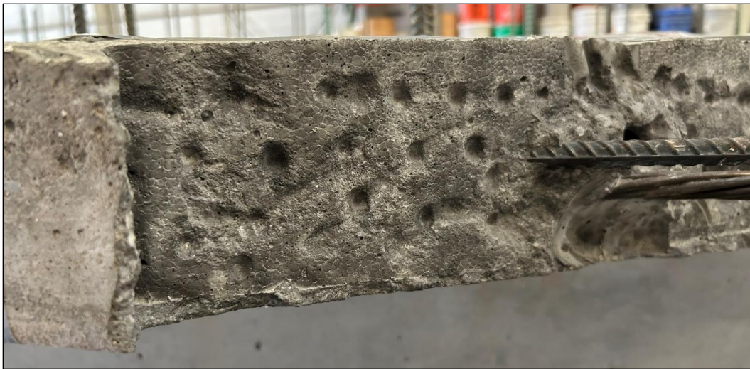
Figure 14. Photo. Top flange repair surface preparation.
