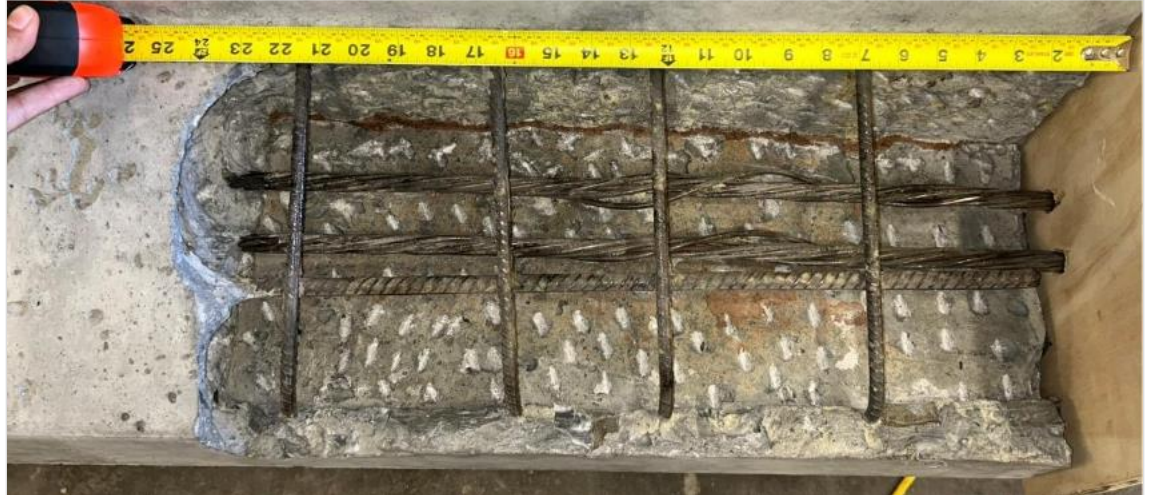
Figure 209. Photo. Repair 4.1LBZ.
