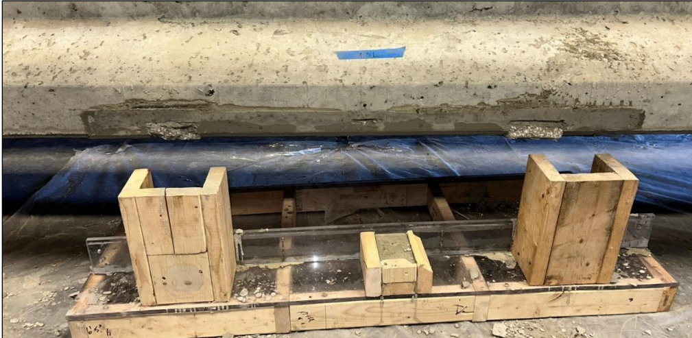
Figure 59. Photo. Repair 4.3LBF after demolding.
