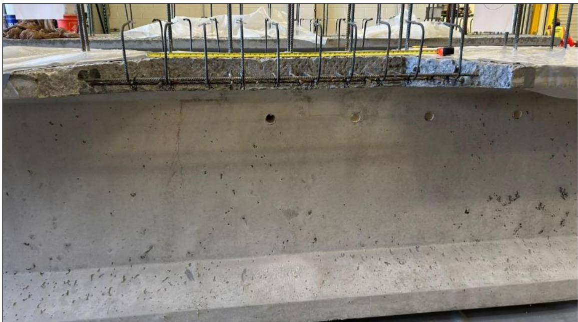
Figure 199. Photo. Repair 1.3RTF.
