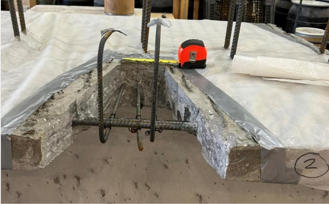
Figure 214. Photo. Repair 4.2RTF.
