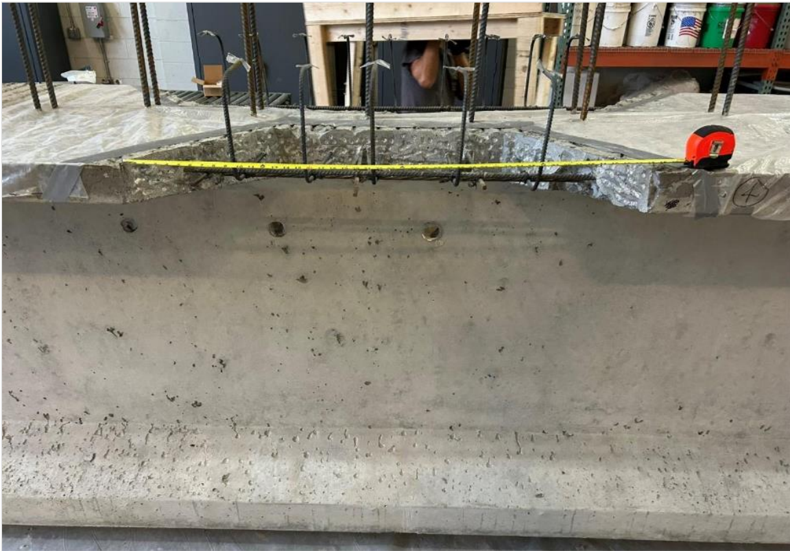
Figure 211. Photo. Repair 4.1RTF.
