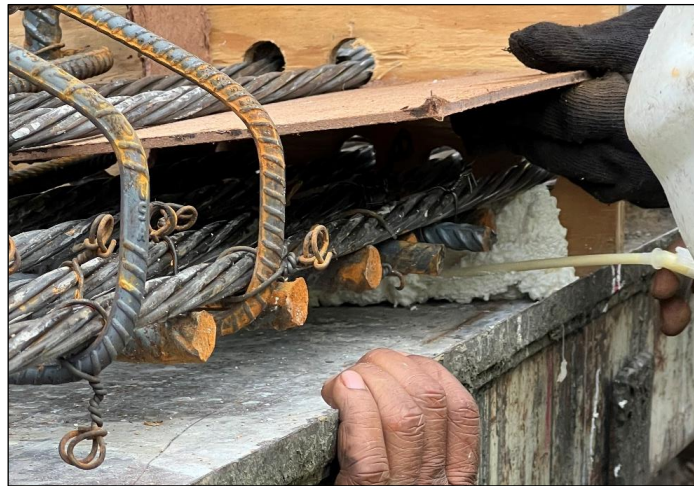
Figure 5. Photo. Typical bearing area block out.
