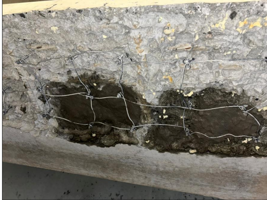
Figure 57. Photo. SikaEmaco 425 Gel Patch non-sag concrete repair mortar on repair 4.3LBF.
