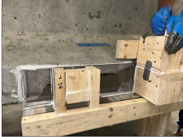
Figure 62. Photo. SCC flowing through the chimney formwork in repair 4.2RBZ.
