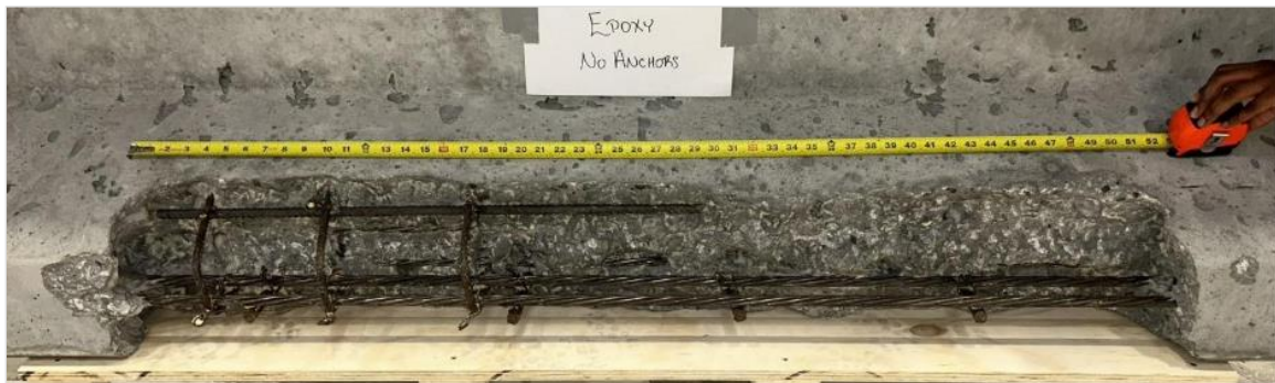
Figure 205. Photo. Repair 3.1RBF.
