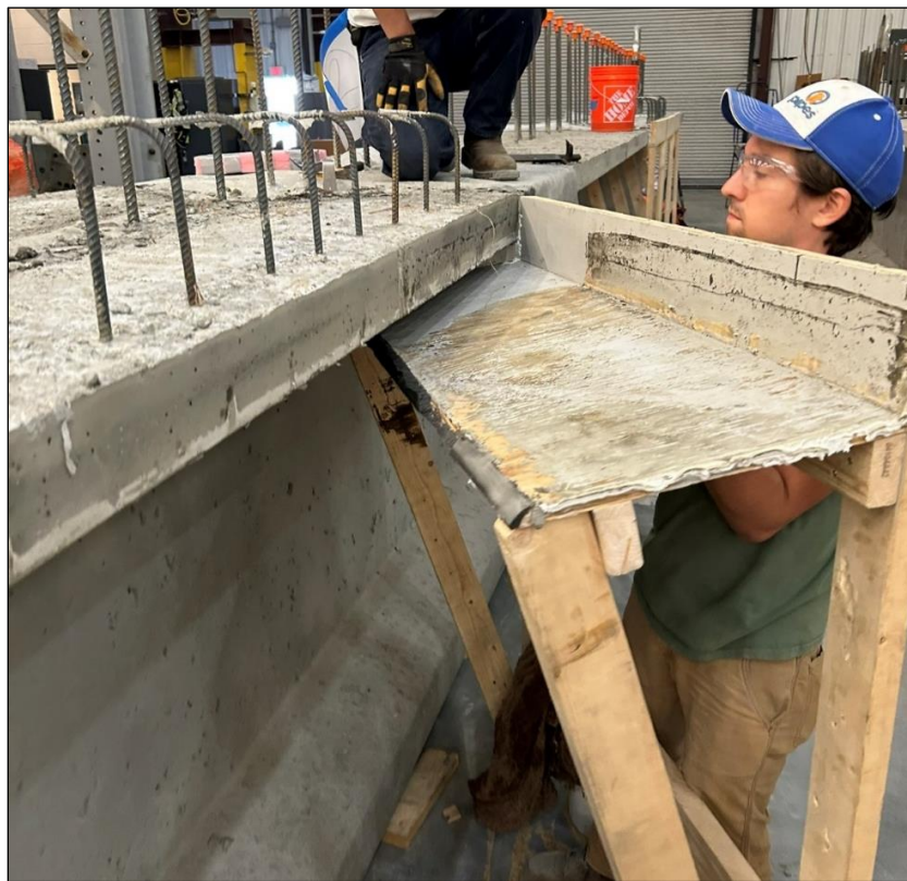
Figure 25. Photo. Demolding of top flange repair.
