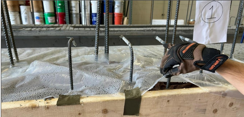
Figure 24. Photo. Concrete curing conditions for top flange repair.
