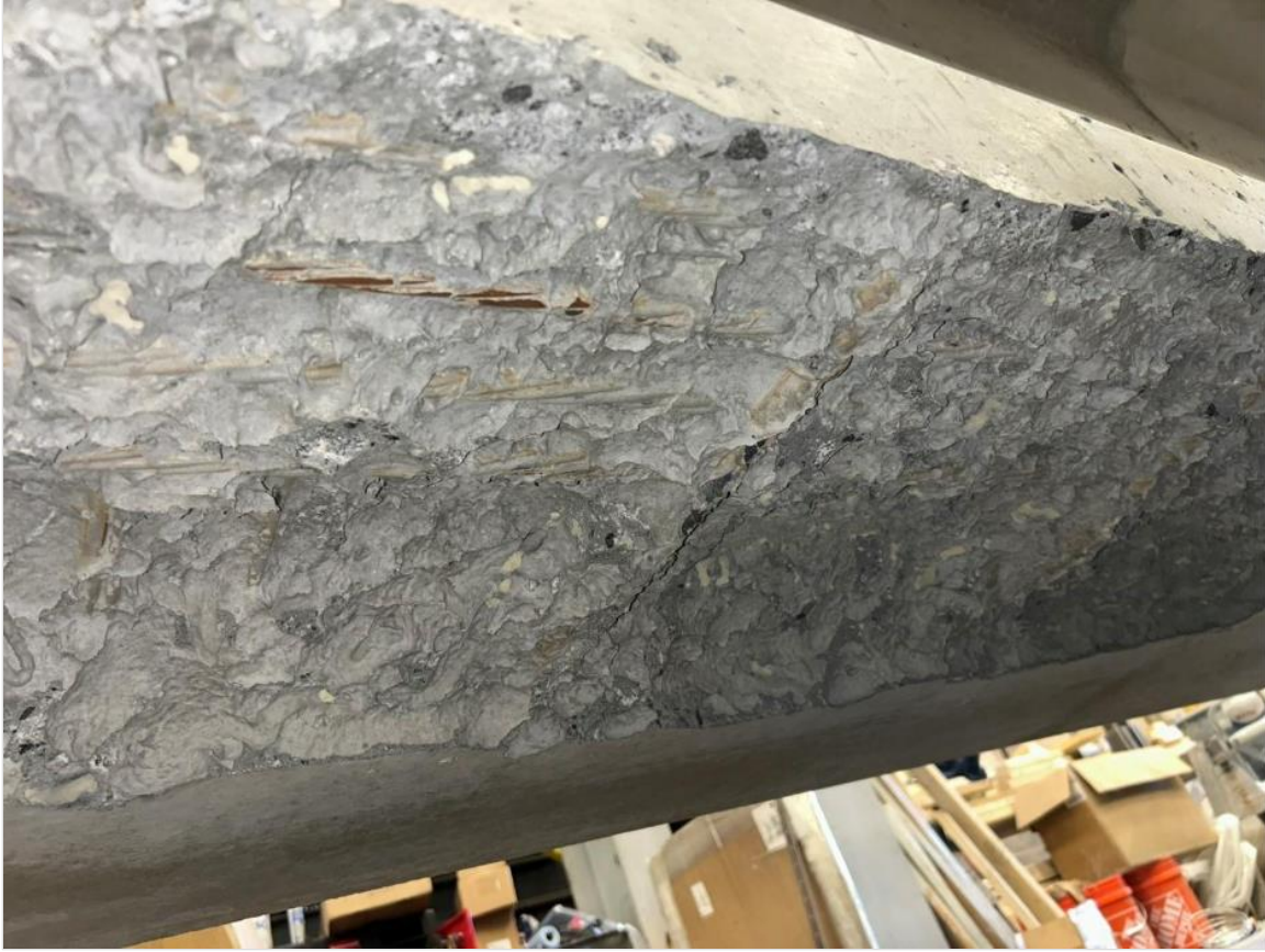
Figure 216. Photo. Repair 4.3LBF.
