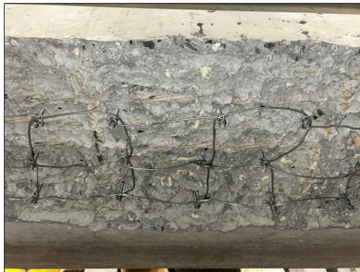
Figure 56. Photo. Stainless steel Tapcon and galvanized wire grid.
