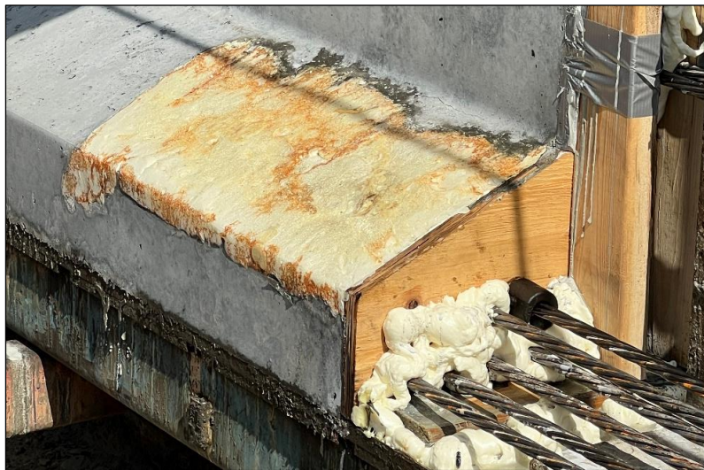
Figure 8. Photo. Typical bottom flange block out after formwork removal (end view).
