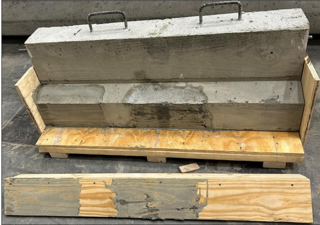
Figure 39. Photo. Bottom flange repair on Mini Girder 1 using the SCC mix.
