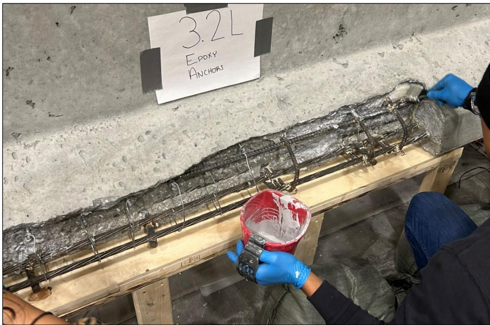
Figure 49. Photo. Coating a bottom flange repair with Sikadur-32 epoxy.
