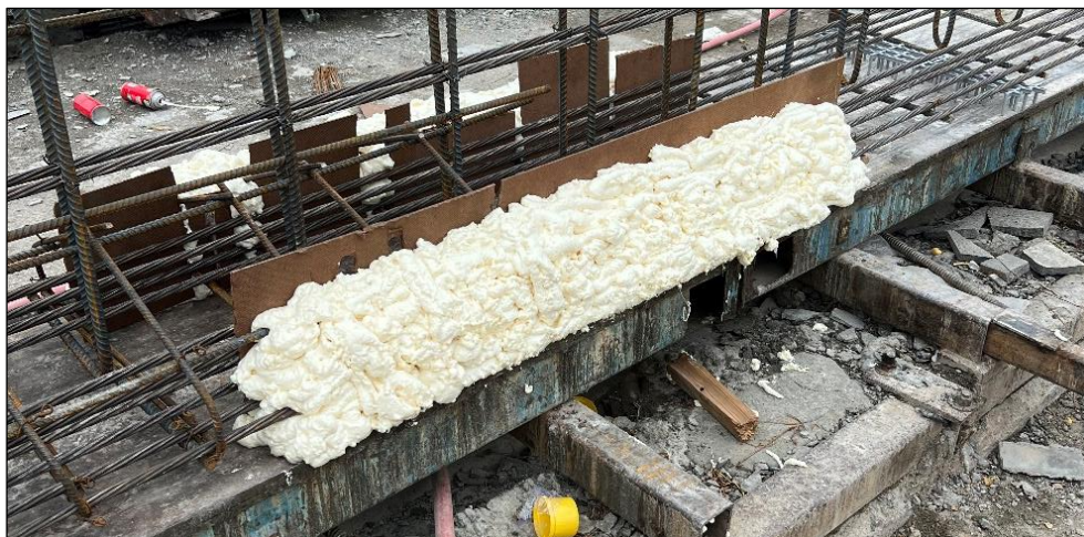
Figure 6. Photo. Typical bottom flange block out.
