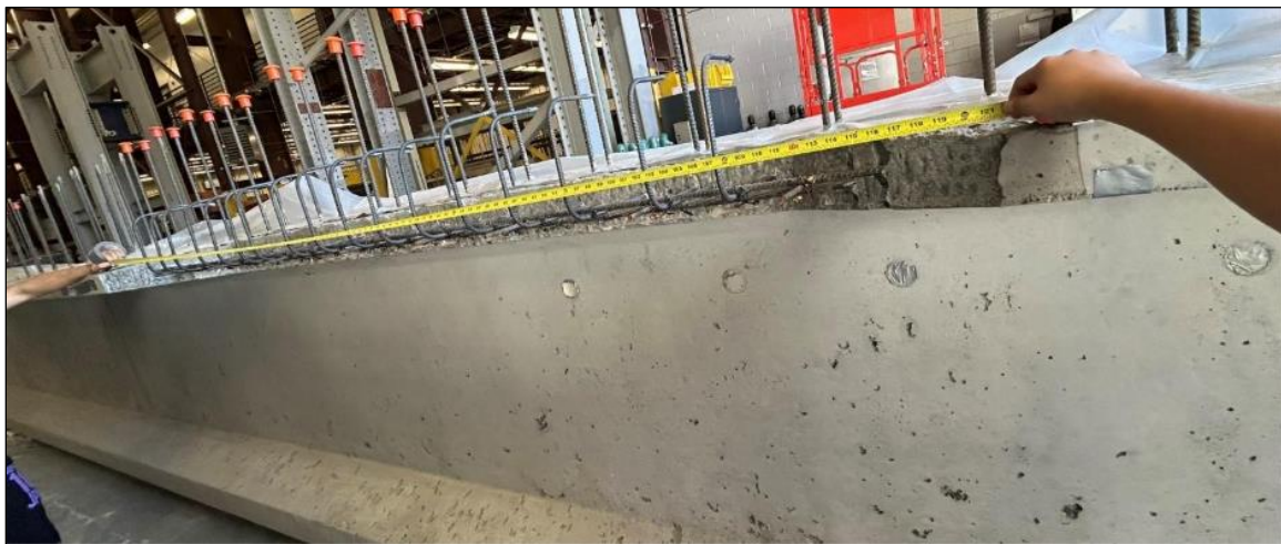
Figure 197. Photo. Repair 1.2LTF.
