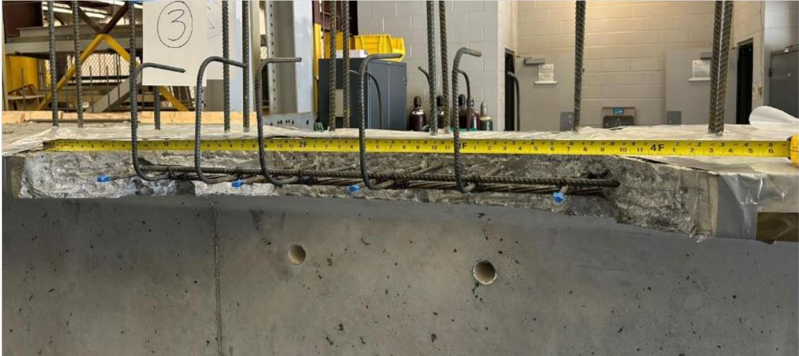
Figure 200. Photo. Repair 2.1LTF.
