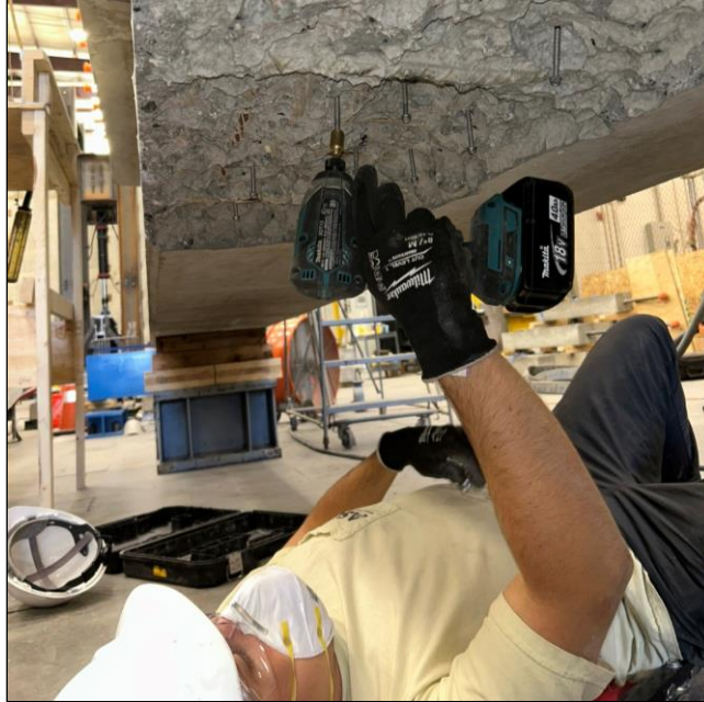
Figure 55. Photo. Installing stainless steel Tapcon into the congested repair.
