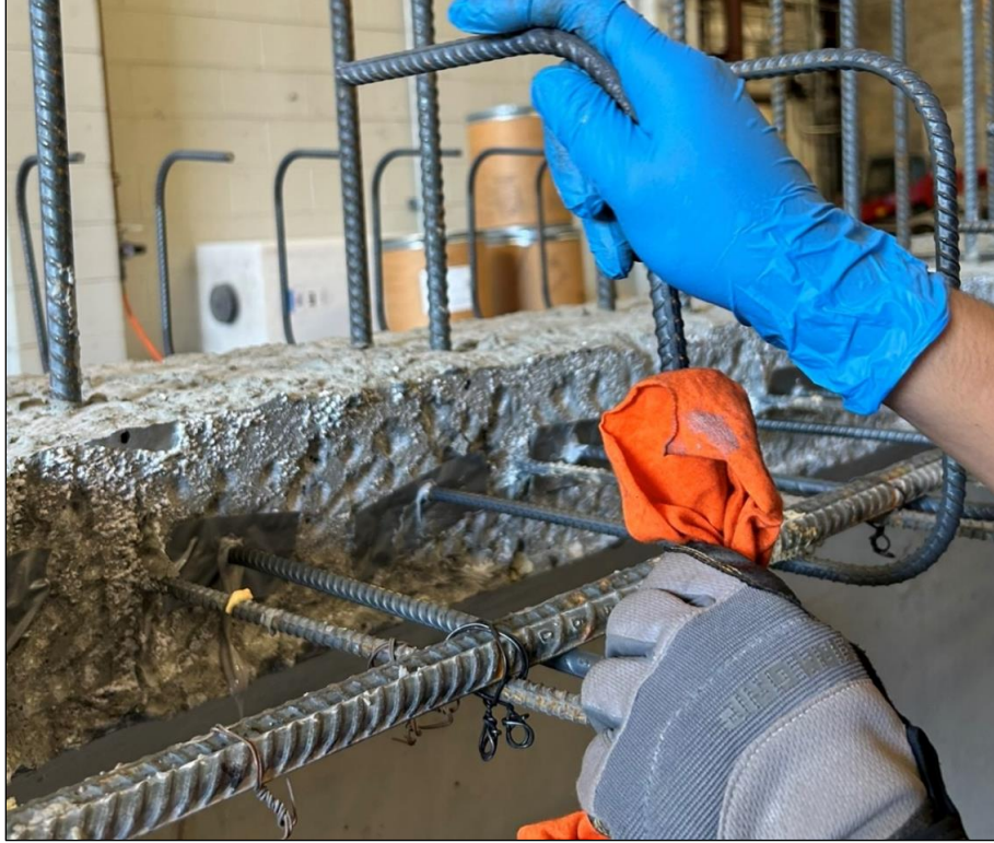
Figure 19. Photo. C-bar installation.
