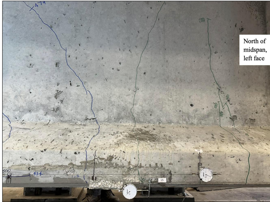
Figure 189. Photo. Test 4.3.F (repair 4.3LBF, 4.3LTF) initial flexural and shear-flexural cracks at 280 kip (left face of girder pictured).
