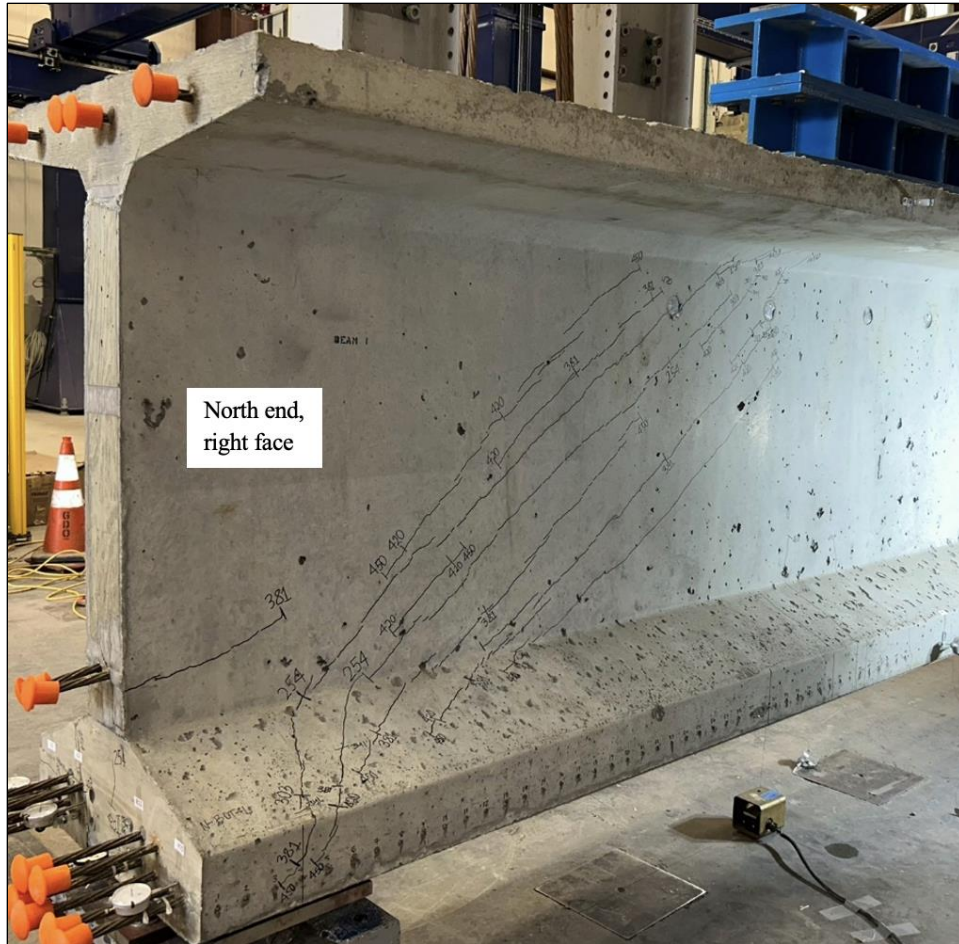
Figure 87. Photo. Test 1.1.S (repair 1.1LBZ) overall crack pattern on original, nonrepaired girder side at 450 kip (right face of girder pictured).
