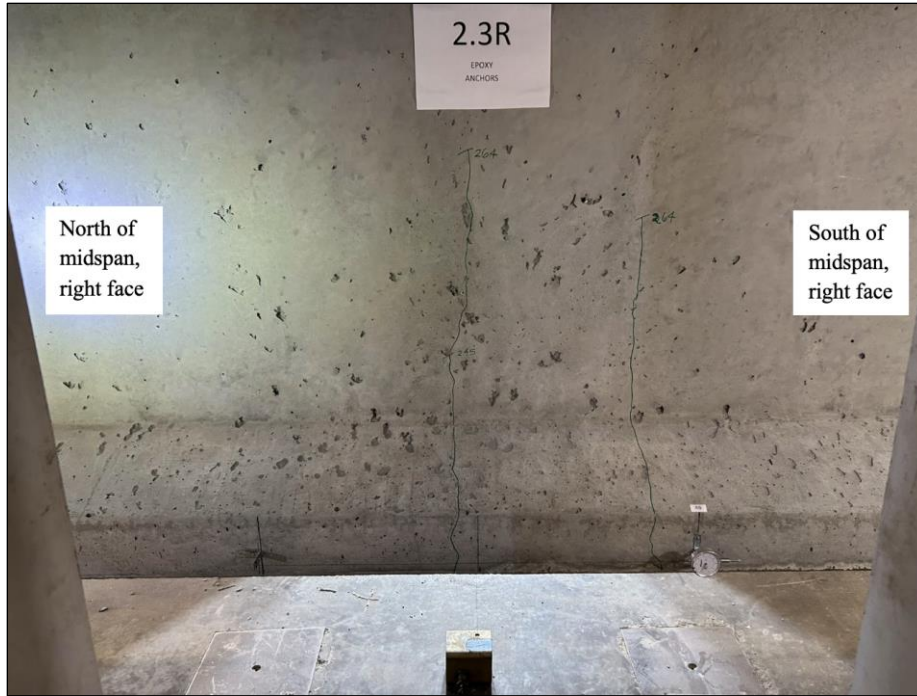
Figure 127. Photo. Test 2.3.F (repair 2.3LTF) flexural cracks at 264 kip (right face of girder pictured).
