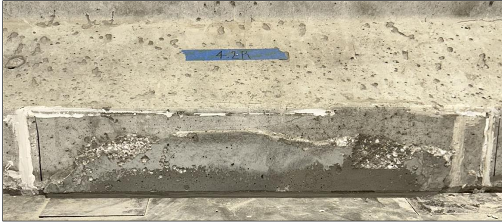
Figure 64. Photo. Repair 4.2RBZ after demolding.
