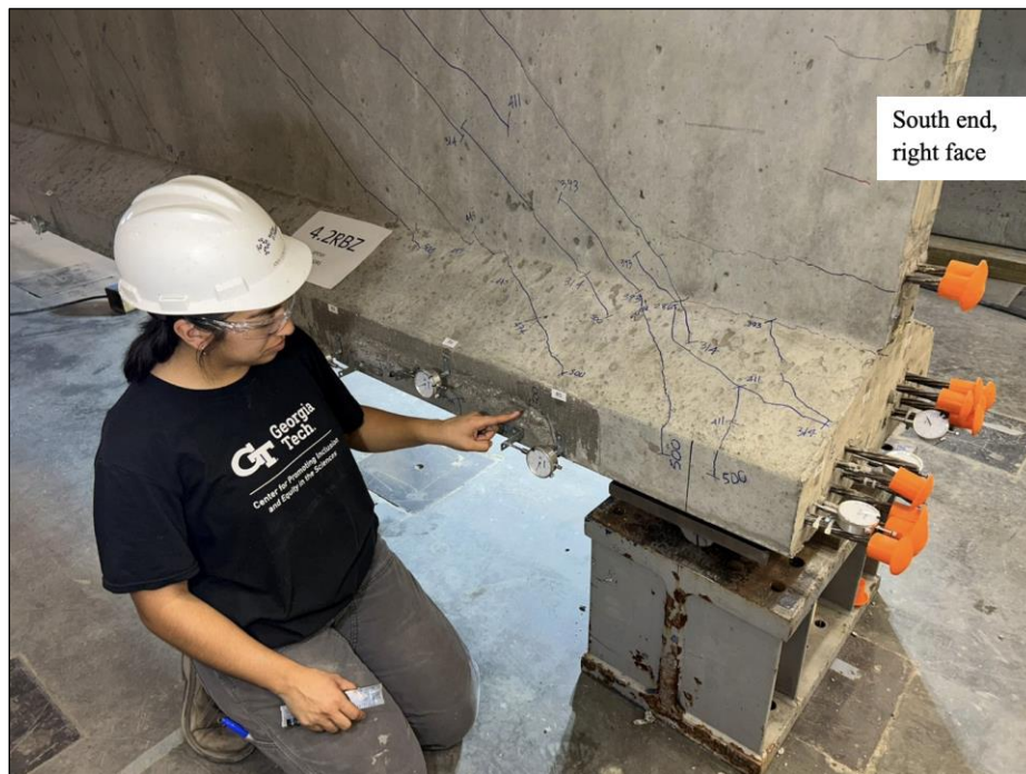
Figure 180. Photo. Test 4.2.S (repair 4.2RBZ, 4.2RTFE, 4.2RTF, 4.2LTF) perimeter cracks at 500 kip with a 0.006-in. repair interface crack measured in dial gauge R5, the outermost strand on the right side, and a strand slip of 0.027 in. measured in dial gauge RS1 (right face of girder pictured).
