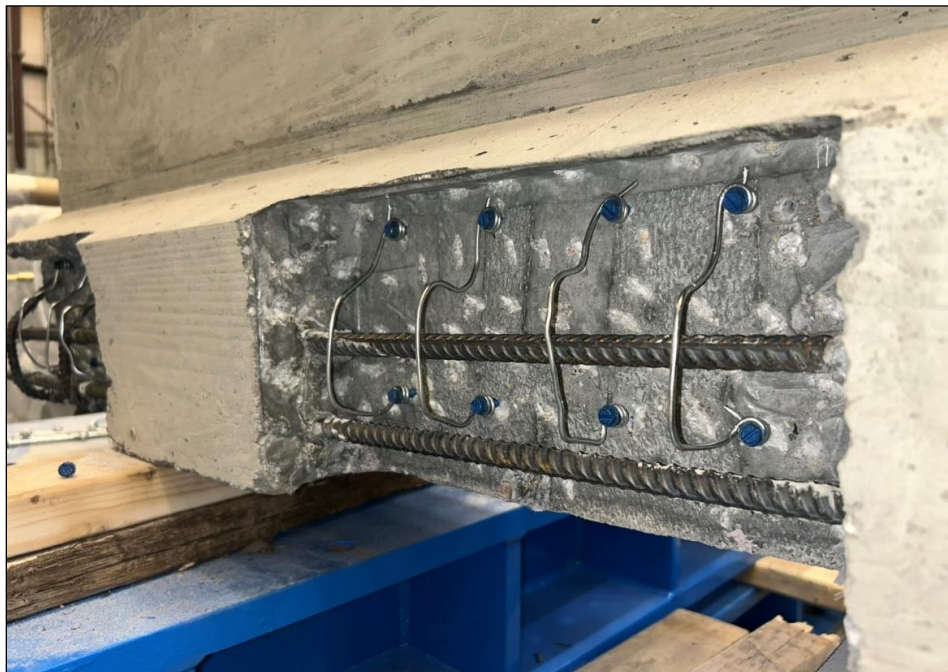
Figure 36. Photo. A 12-gauge wire installation studied as an alternate to reinforcing bars originally recommended by MNL-137.
