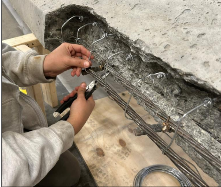
Figure 45. Photo. Installing 12-gauge galvanized wire.
