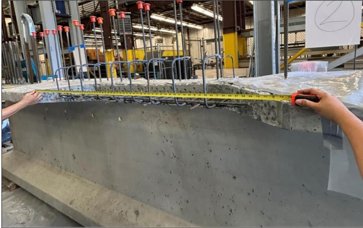
Figure 198. Photo. Repair 1.3LTF.
