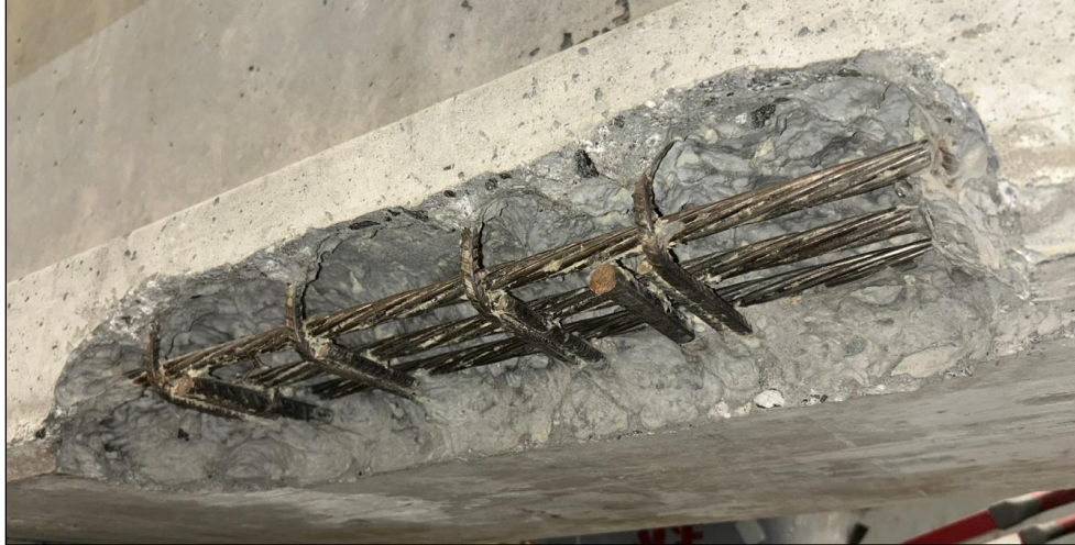
Figure 60. Photo. Repair 4.2RBZ with rebar congestion.
