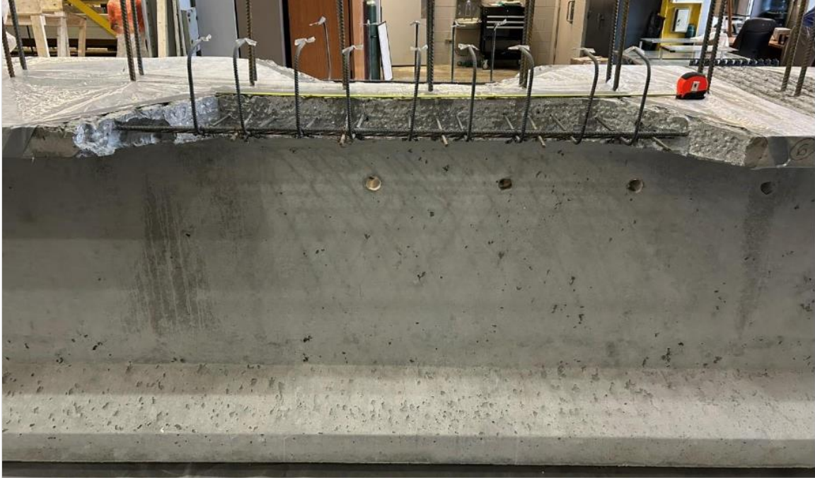
Figure 210. Photo. Repair 4.1LTF.
