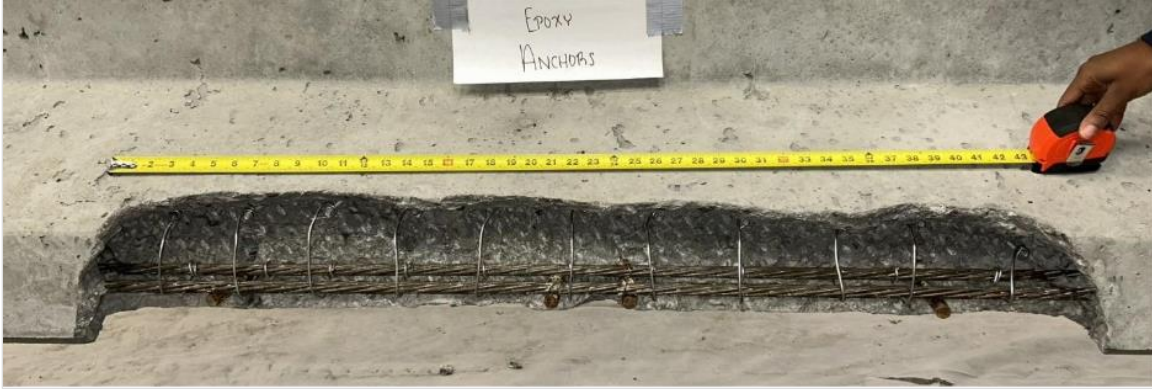
Figure 207. Photo. Repair 3.3LBF.
