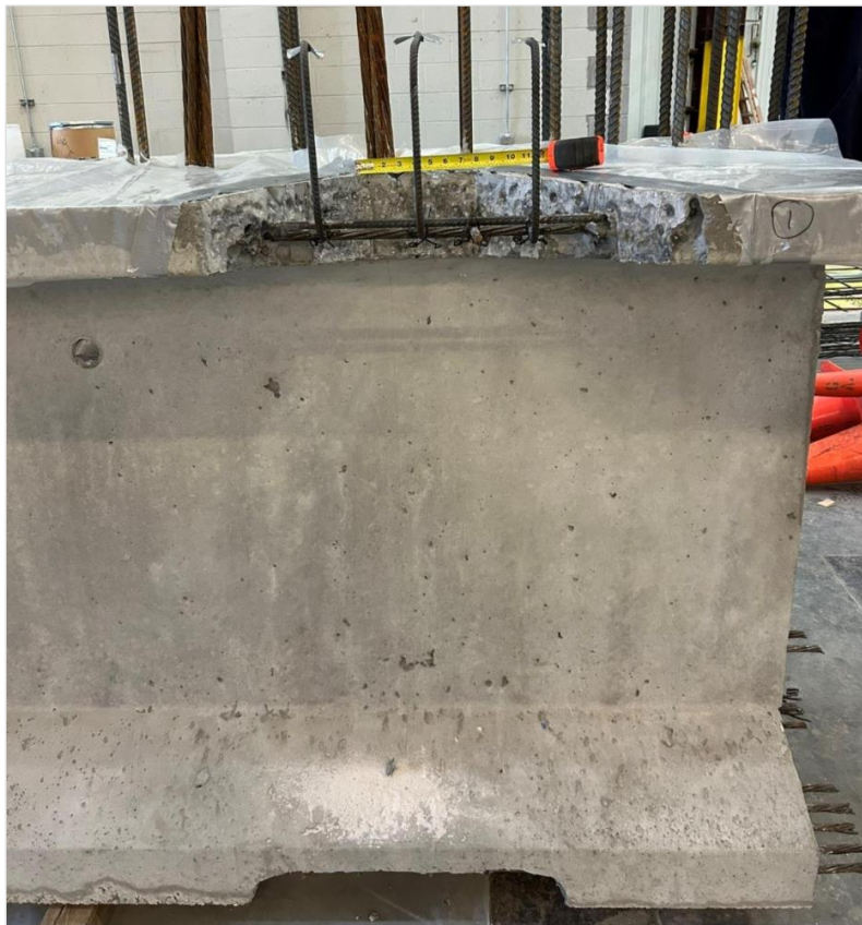
Figure 215. Photo. Repair 4.2RTFE.
