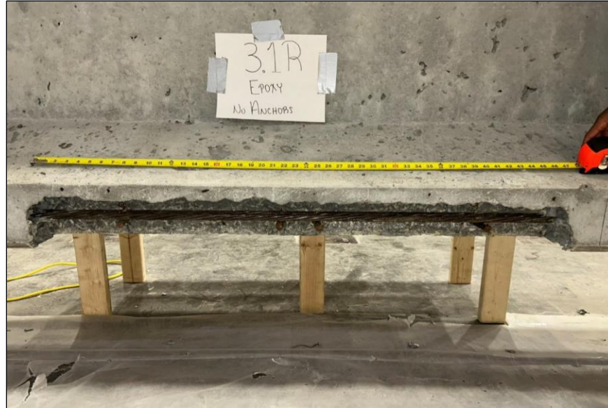
Figure 47. Photo. Bottom flange repair 3.1RBF with no post-installed anchors.
