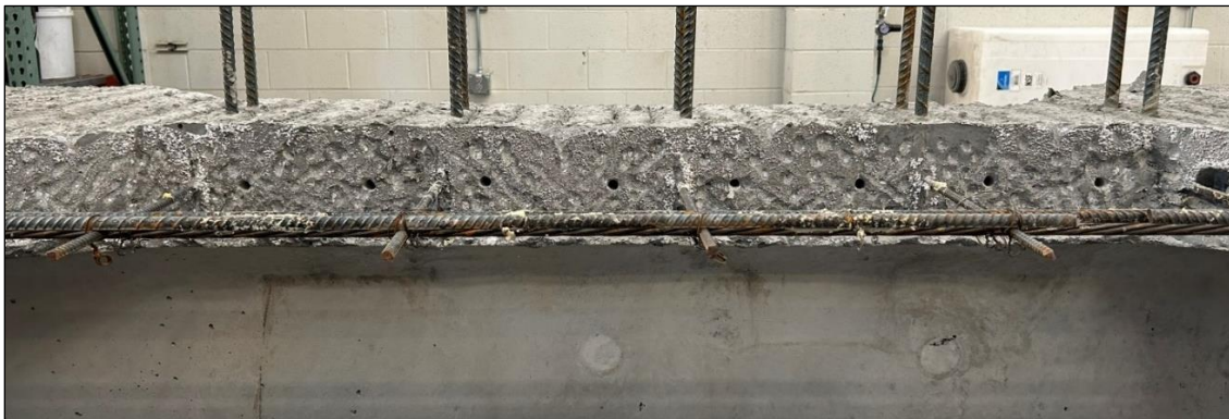
Figure 4. Drilled holes for c-bars.
