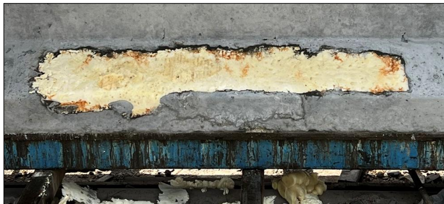
Figure 9. Photo. Typical bottom flange block out after formwork removal (top view).
