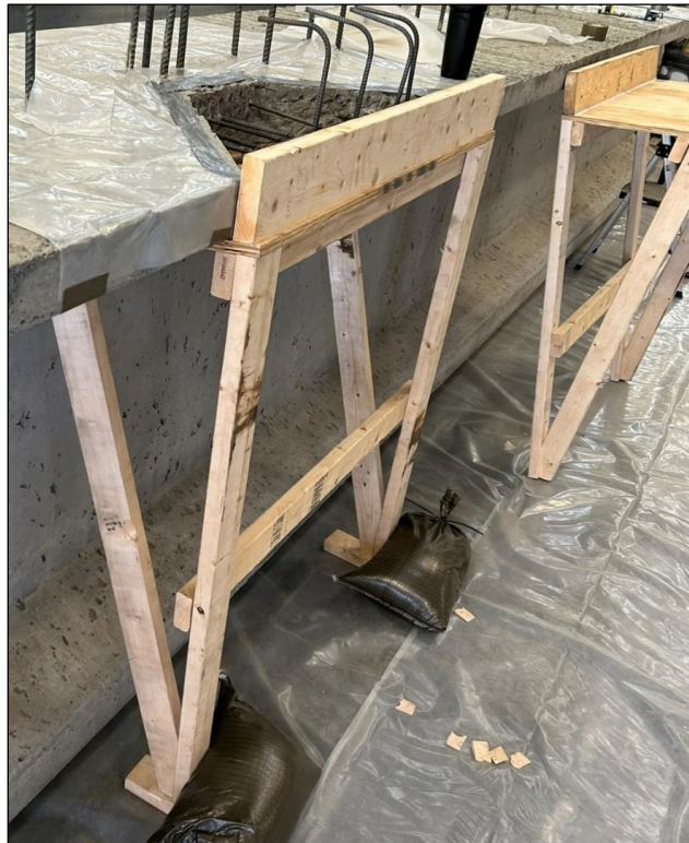
Figure 20. Photo. Top flange repair formwork.
