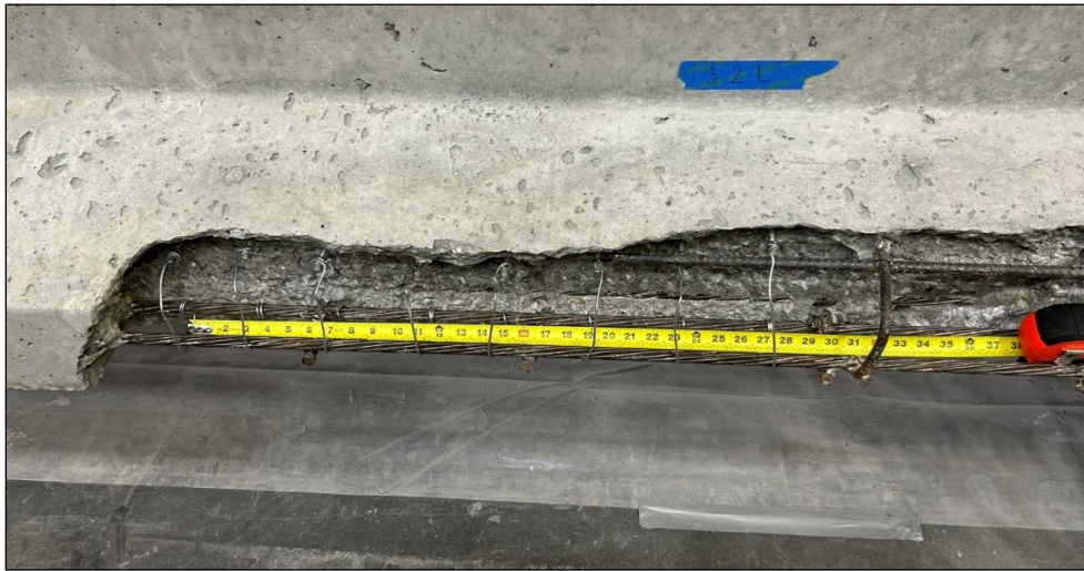
Figure 46. Photo. Post-installed steel anchors and wire in a bottom flange repair.
