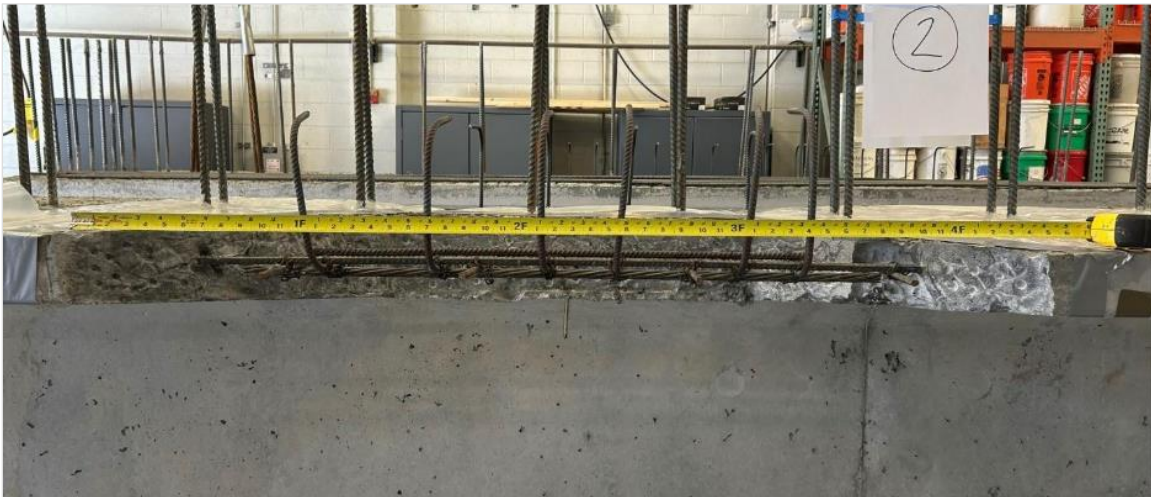
Figure 201. Photo. Repair 2.1RTF.
