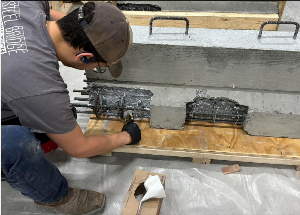
Figure 37. Photo. Installation of the epoxy bonding agent.
