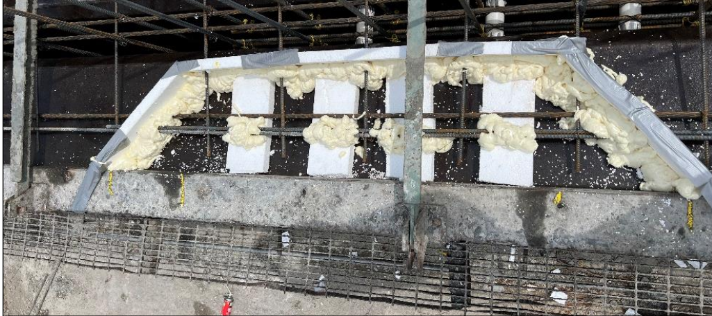
Figure 7. Photo. Typical top flange block out.
