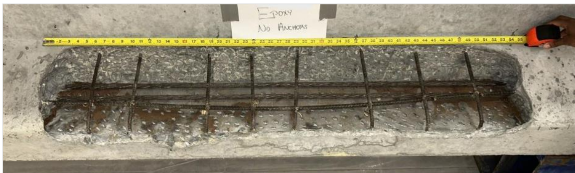
Figure 206. Photo. Repair 3.2RBF.
