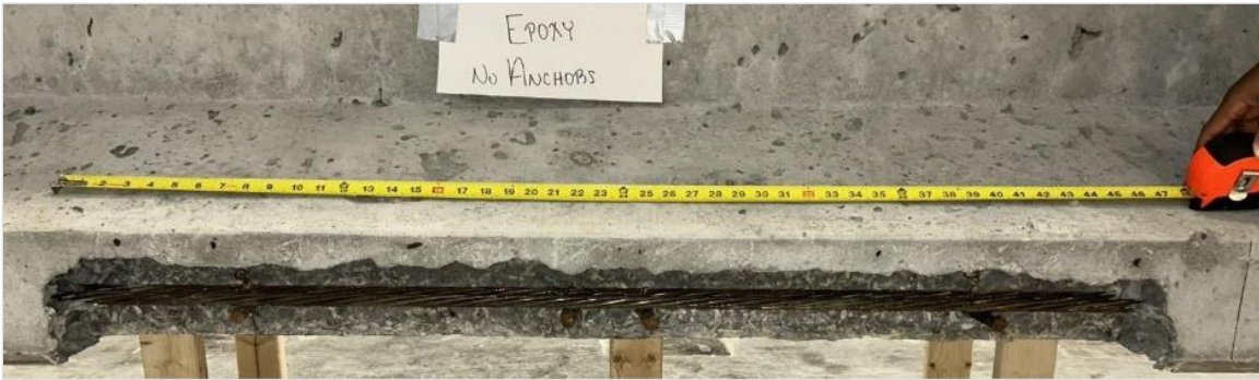
Figure 208. Photo. Repair 3.3RBF.
