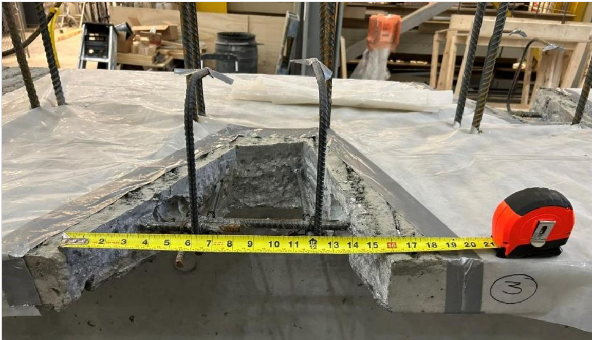
Figure 213. Photo. Repair 4.2LTF.
