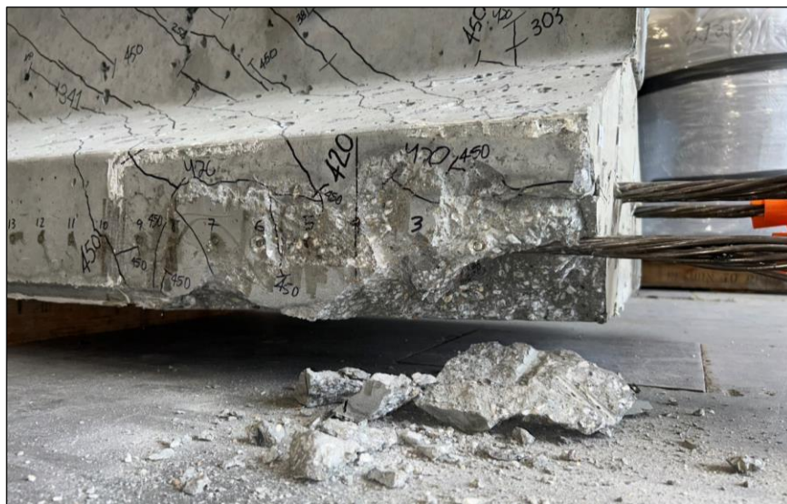
Figure 88. Photo. Test 1.1.S (repair 1.1LBZ) residual strength test using a sledgehammer.
