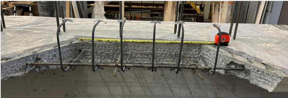
Figure 217. Photo. Repair 4.3LTF.
