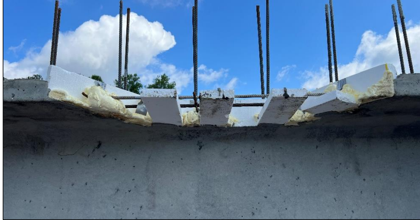
Figure 10. Photo. Typical top flange block out after formwork removal.
