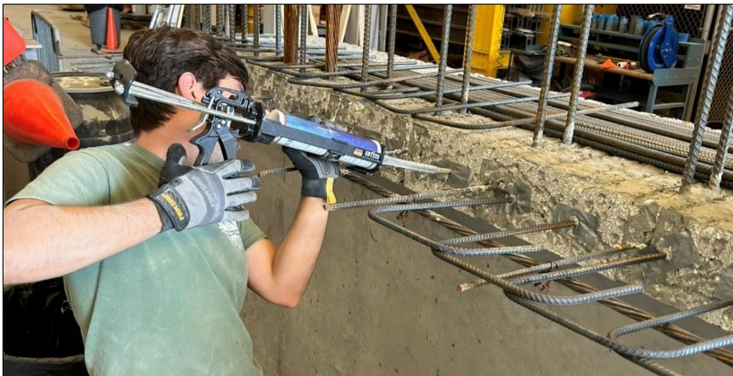
Figure 18. Photo. Insertion of two-part Unitex Pro-Poxy 300 into cleaned drilled holes.
