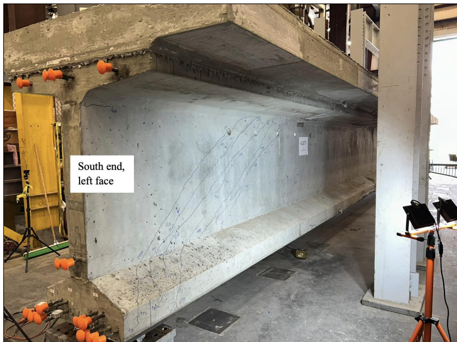
Figure 182. Photo. Test 4.2.S (repair 4.2RBZ, 4.2RTFE, 4.2RTF, 4.2LTF) final shear cracks on top flange repaired face at 500 kip (left face of girder pictured).
