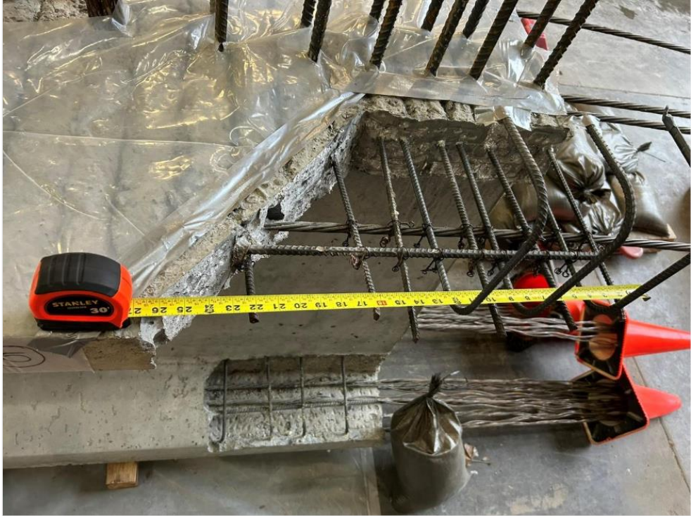
Figure 218. Photo. Repair 4.4LTF.
