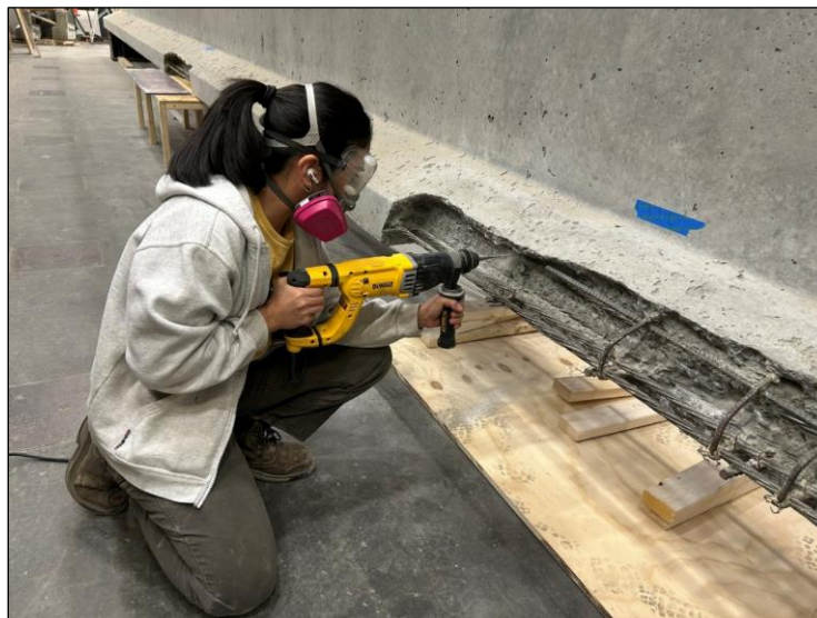
Figure 44. Photo. Drilling pilot holes for stainless steel Tapcon concrete anchors.
