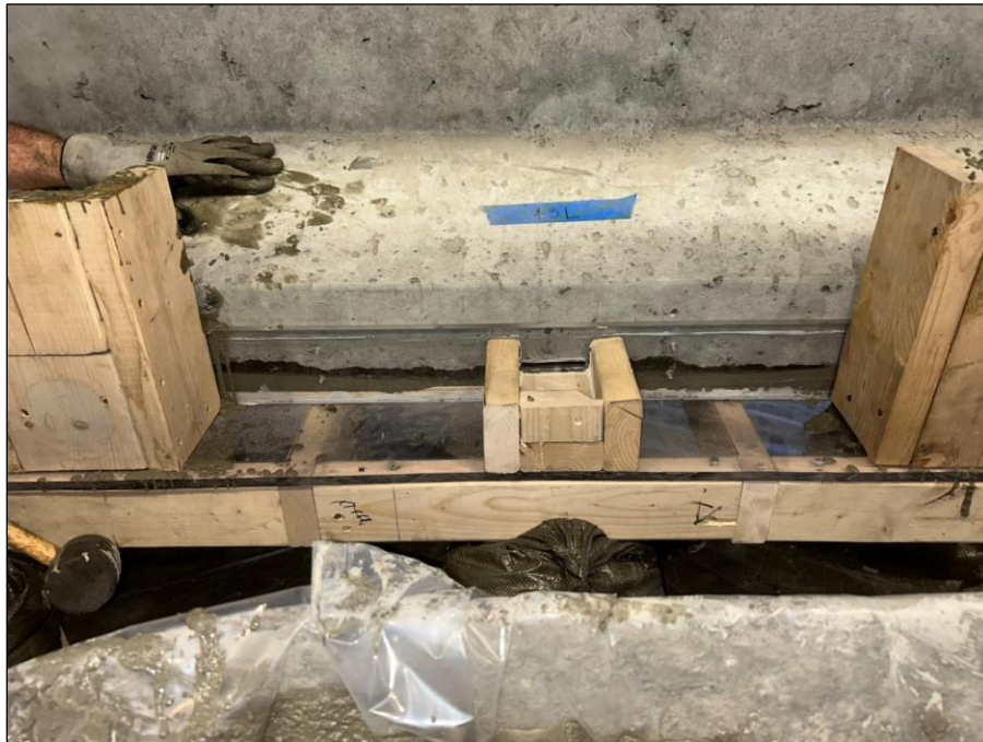
Figure 58. Photo. Repair 4.3LBF during concrete casting.
