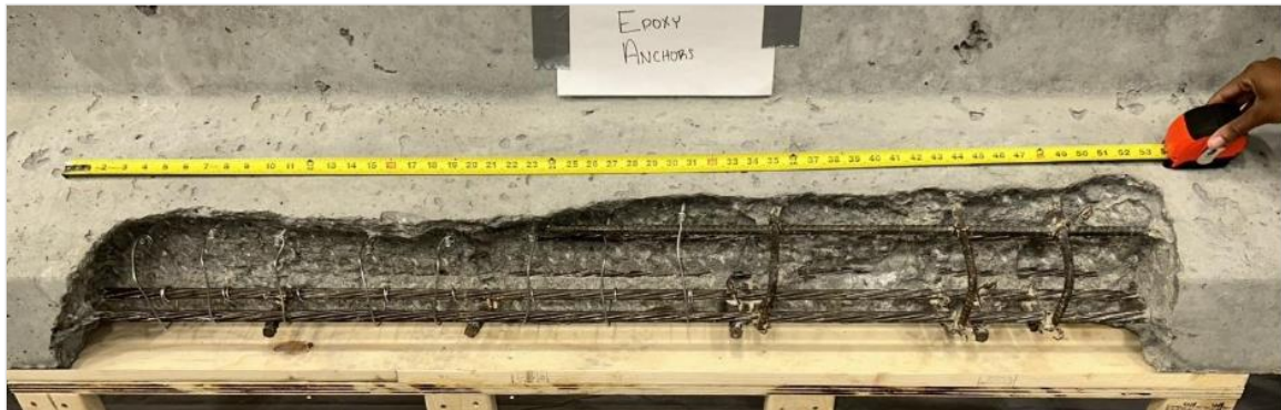
Figure 204. Photo. Repair 3.1LBF.
