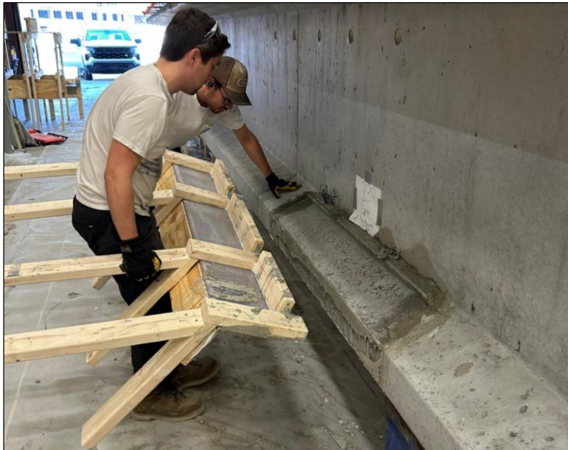
Figure 53. Photo. Demolding of repair 3.3RBF.
