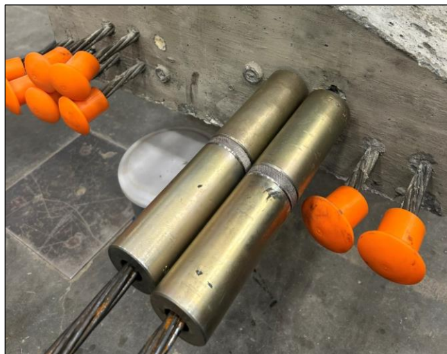
Figure 70. Photo. Splice chucks used to extend strands through the abutment.
