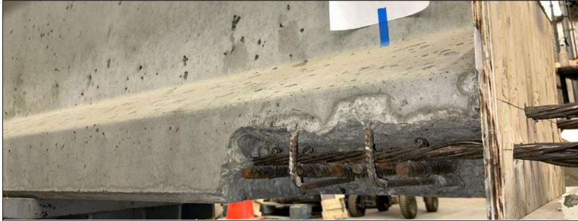
Figure 196. Photo. Repair 1.1LBZ.
