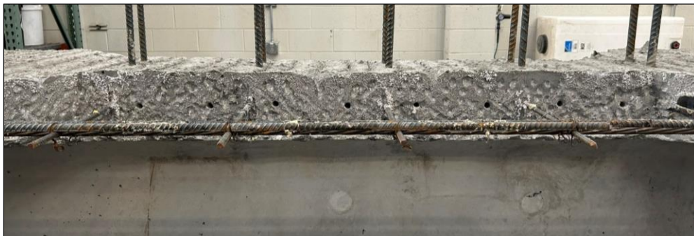
Figure 17. Photo. Drilled holes for c-bars.
