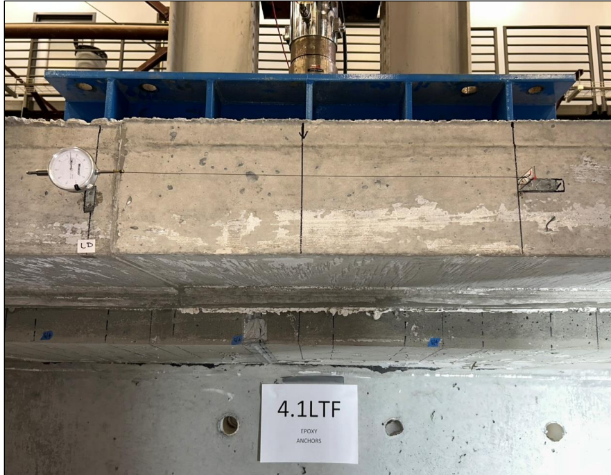
Figure 163. Photo. Test 4.1.S (repair 4.1LBZ, 4.1RTF, 4.1LTF, 4.4LTF) general test setup (left face of girder pictured).
