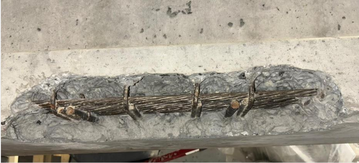
Figure 212. Photo. Repair 4.2RBZ.
