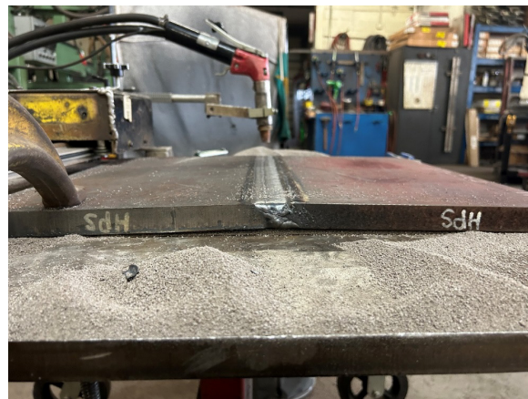
Step 4: Perform repair weld using SAW.
