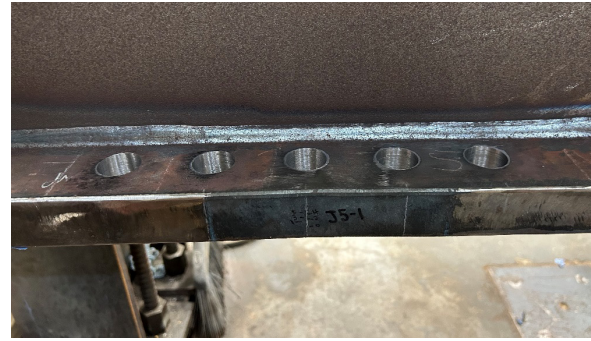
(b) Bolt Holes Drilled in Flange
