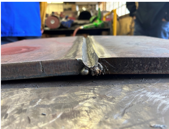
Step 3: Excavate “defect” by arc gouging and grinding.
