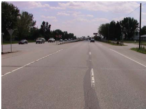
d) Suburban divided with median barrier
