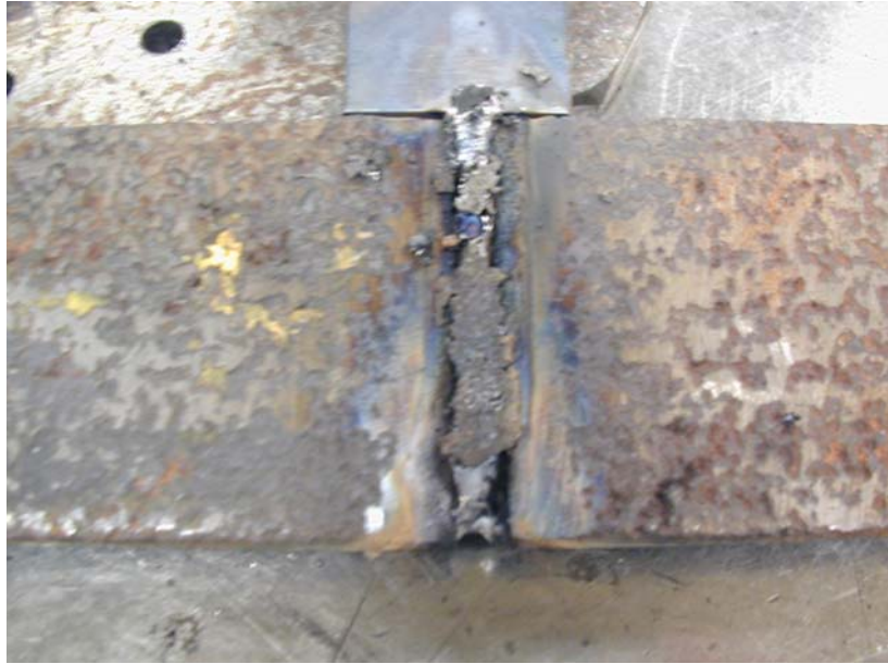
Figure D.3 Surface Impurities or Scale on Surface of Weld
