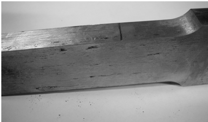
Figure 5.2 Typical Surface Appearance of Wrought Iron in Many Existing Bridges
