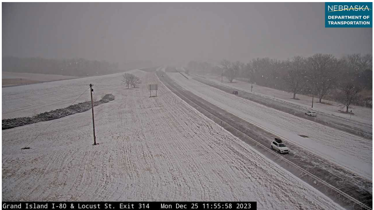
Figure 4.22 Grand Island, Case 3 winter maintenance performance dashboard (top) and Grand Island segment, Case 3 traffic camera image at Exit 314 at 1155 CST on 25 December 2023.
