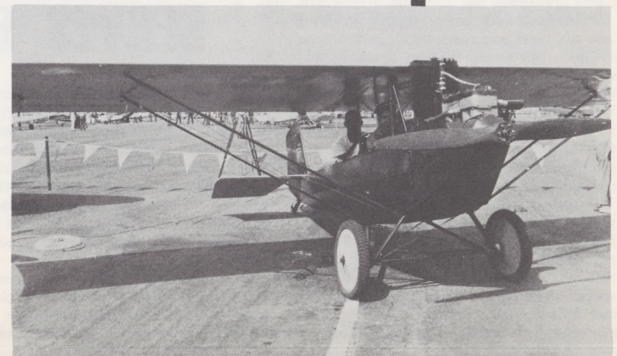
"Now, if we can get this thing started—we're off." (Note the Model "B" modified Ford engine, complete with radiator.)
