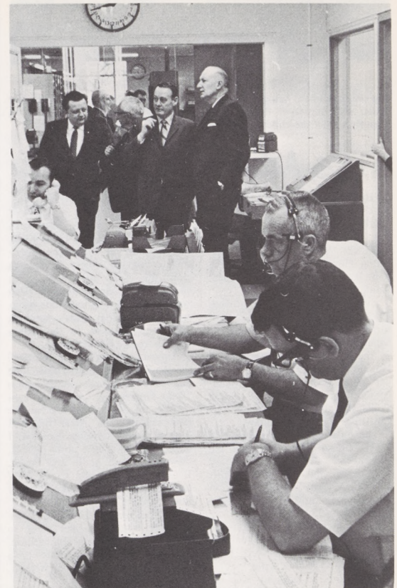
As (from left) Tom Johnson, Roger Alexander and John Marquardt perform flight service specialist duties, others look over the new installation. In the background are Al Hinz, Chicago FSS; Jack Brazee, Joliet FSS, retired; George Biehl, Chicago FSS; and Paul E. Cannom, Chicago Area Manager.
