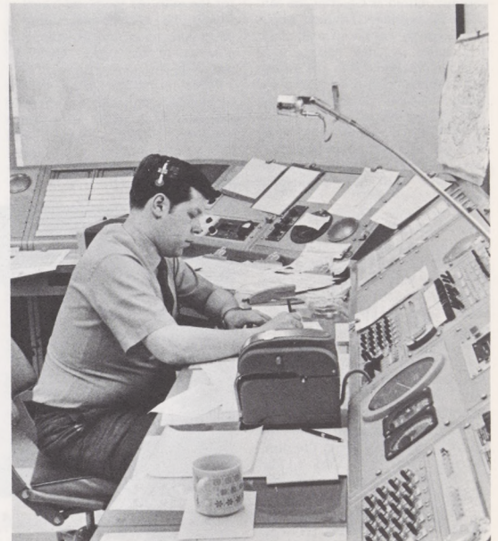
One of the four air-to-ground radio consoles installed in a special sound proof room at the newly commissioned station is operated by Dave Phillips of the Chicago FSS.
