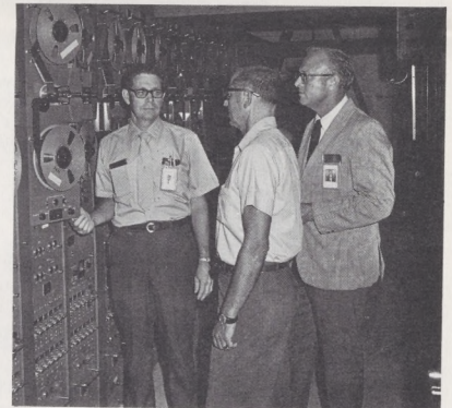
Recording equipment at the Memphis Center is checked over by Charles McCormick (left), communications unit leader, Russ Hillen (center), electronics technician and Bill Edwards, systems engineer.
