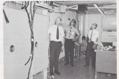
Inside of transportable ASR-7 radar building is inspected at Dallas by (from left) Dan Watson, Texas Instruments engineer and Al Hockstein and Earl Gray, FAA Quality and Reliability Representatives.
