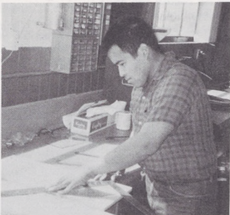
Roy Eskalida of the Gulkana sub-sector repairs a window of one of the housing units.
