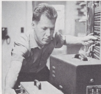
Trouble-shooting a circuit in the Big Delta FSS is Electronics Technician Joe Brunner.
