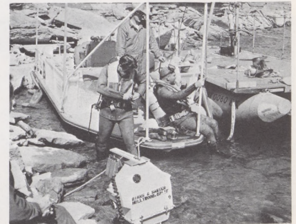
One of the agency's most unusual vehicles is this 21-foot Hydrodyne boat used by the Civil Aeronautical Institute at the Aeronautical Center to conduct studies of flotation equipment and means of escape from ditched and submerged aircraft. Here, divers and photographers prepare to install underwater apparatus used in photographing impact tests of a flotation device which will be dropped from nearby cliffs.
