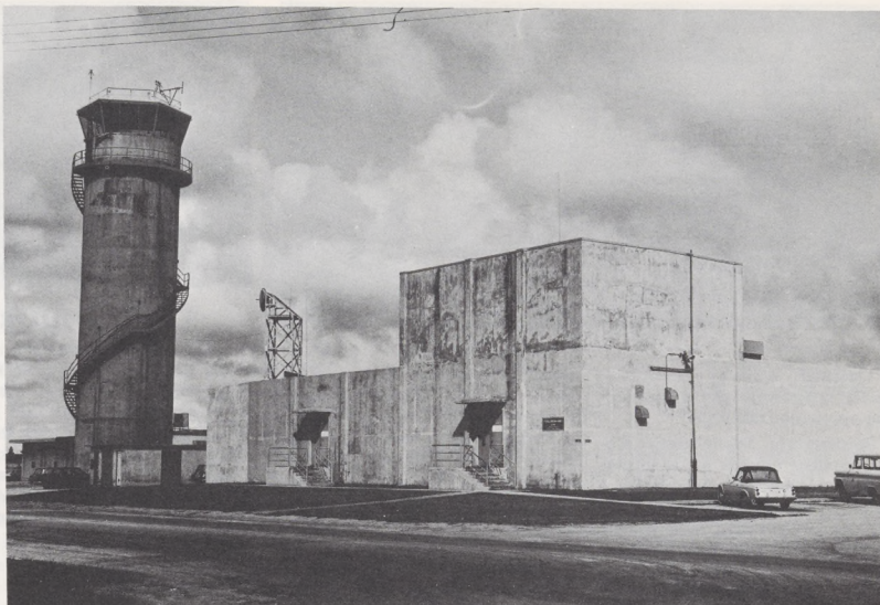
Outer walls of the Guam Center/RAPCON (CERAP) are built to withstand the devastating storms that now and then plague the usually lush, peaceful Pacific island.
